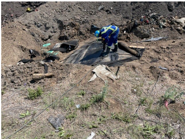
Repair in Progress
