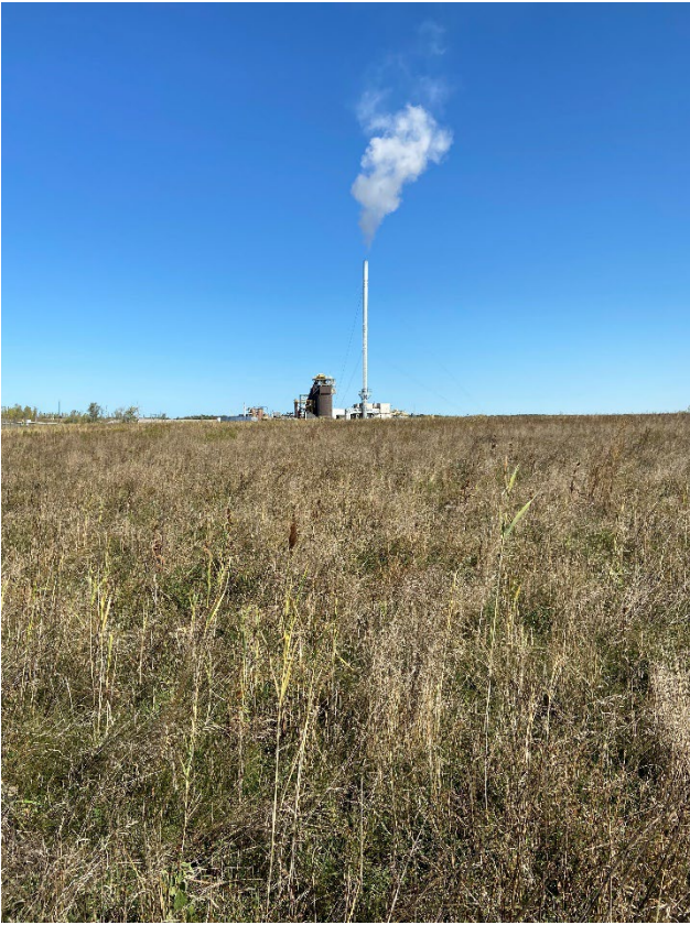
Photo 11: Location for the new Site S8, south of the smoke stack.
