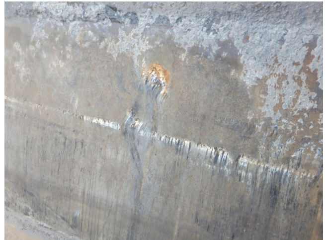
(Photo 4) Scraping On The Wall
