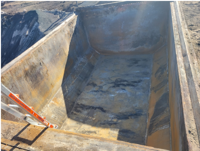
(Photo 3) Pit Overview
