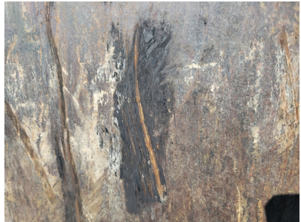
(Photo 6) Scraping On The Wall (2)
