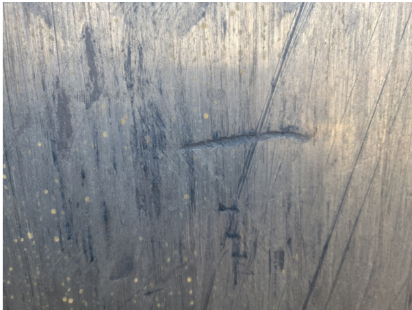
(Photo 5) Scraping On The Wall
