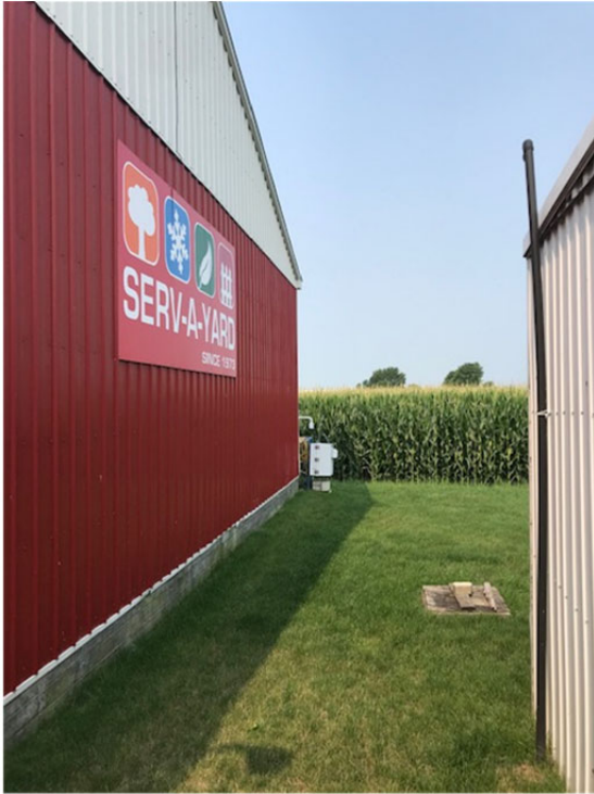
From East Looking West
