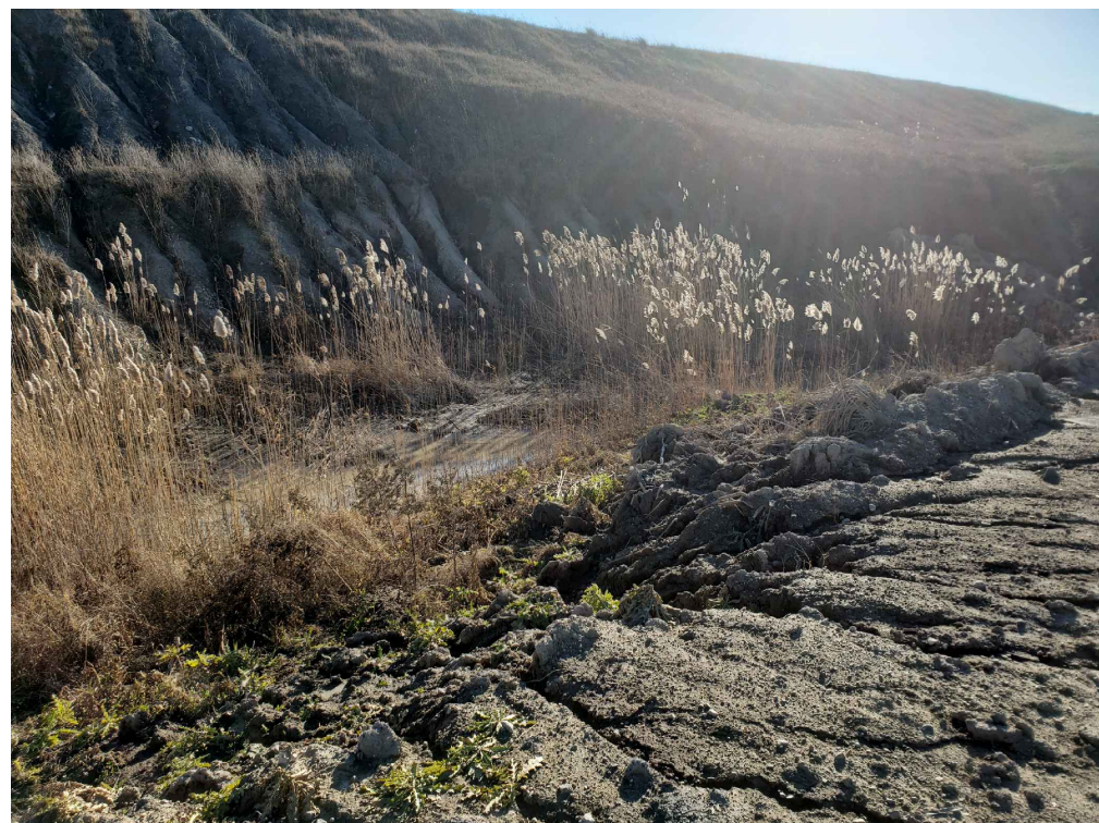
11 EROSION CHANNELS AND SEDIMENTATION ALONG EAST PERIMETER DITCH Fig 4A
