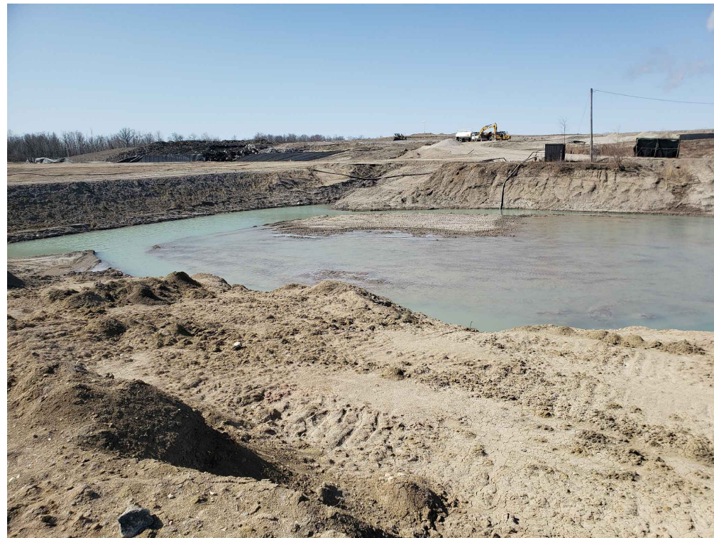
17 FORMER EAST SURFACE WATER POND - ACTIVE DEWATERING FOR CELL 20-1 Fig 4A
