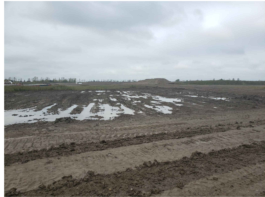
10 NORTHEAST CORNER OF THE SITE LOOKING WEST Fig 4A
