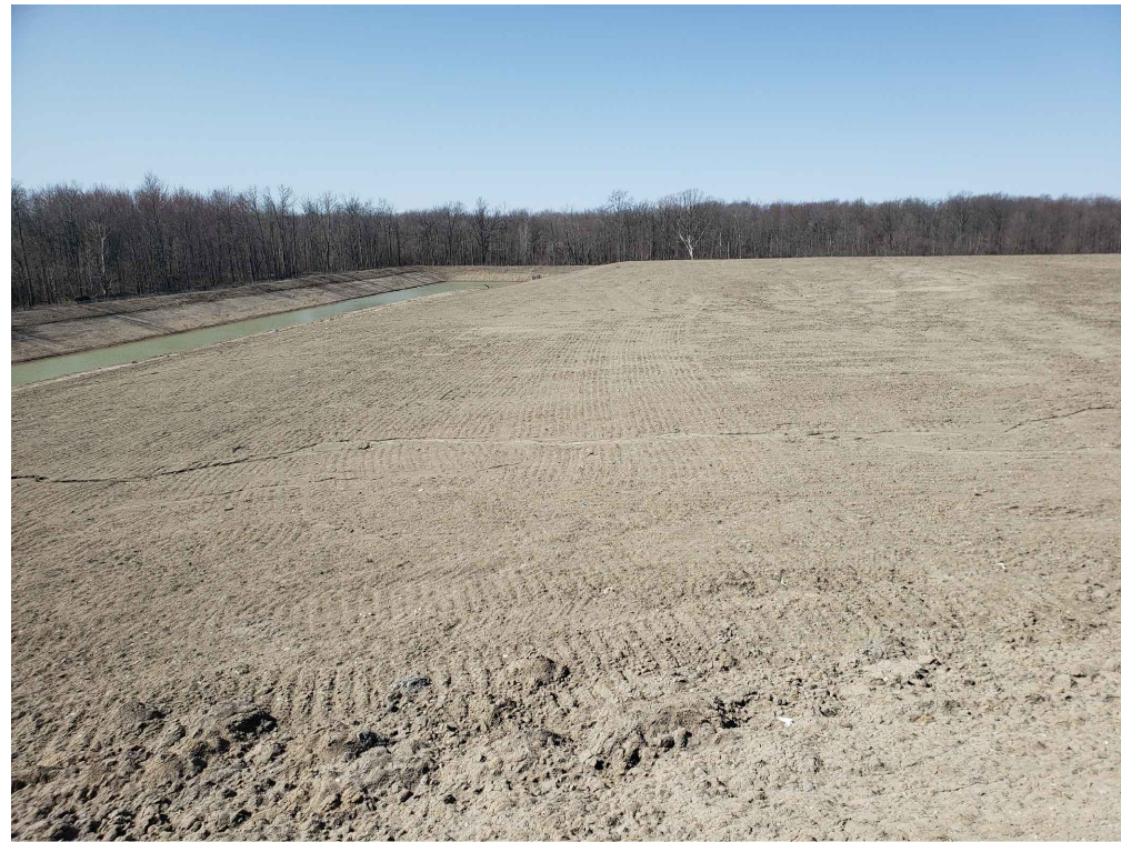
5 FINAL COVER - TOPSOIL PLACEMENT CELL 19-1 Fig 3A
