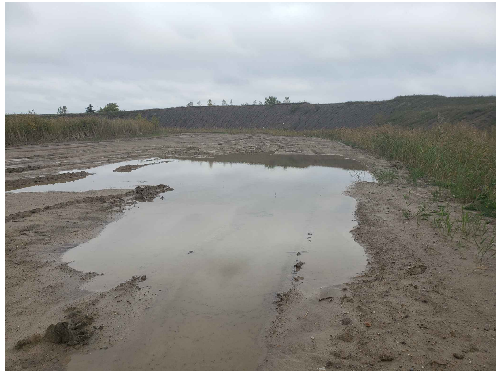
11 EROSION CHANNELS ALONG EAST PERIMETER BERM Fig 4A
