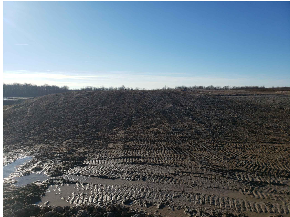
3 CELL 19-3A AREA INTERIM COVER Fig 3A
