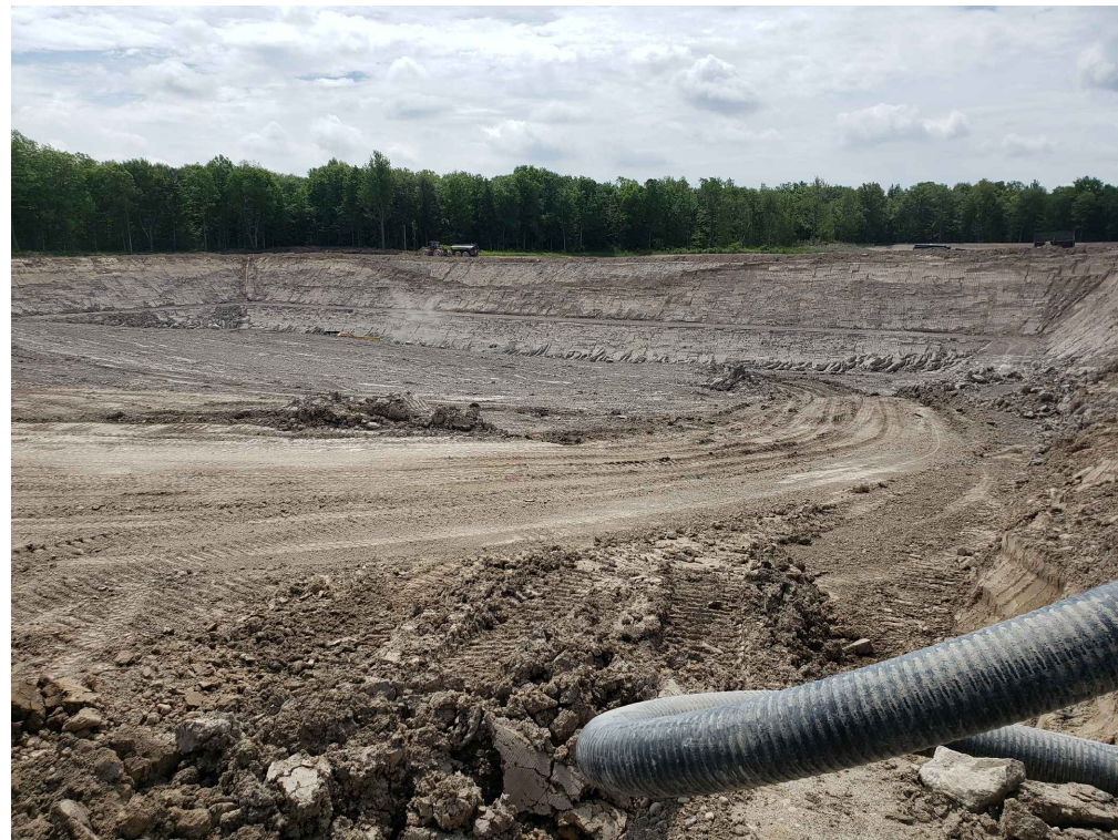
17 Fig 4A FORMER EAST SURFACE WATER POND - CELL 20-1 EXCAVATION
