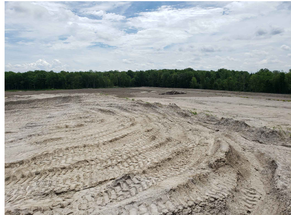
8 CELL 19-2 CLAY STOCKPILE AND INTERIM COVER Fig 3A
