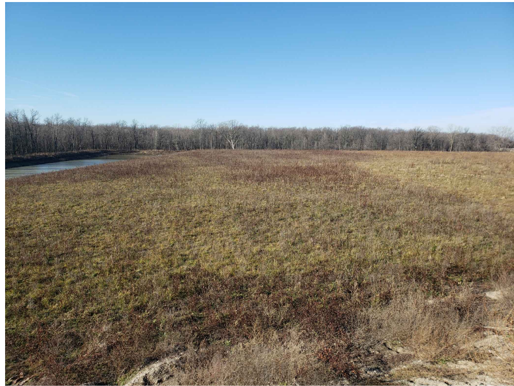
5 FINAL COVER - TOPSOIL PLACEMENT CELL 19-1 Fig 3A
