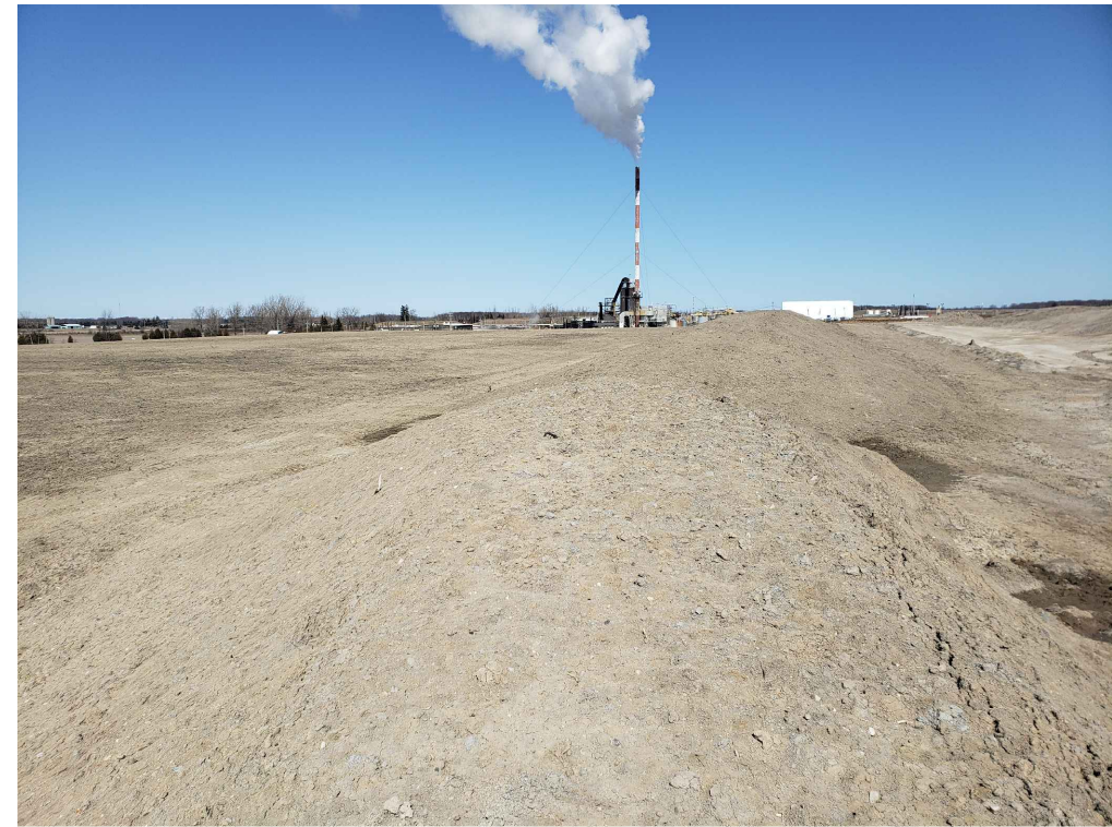
6 FINAL COVER - TOPSOIL PLACEMENT CELL 19-1 Fig 3A
