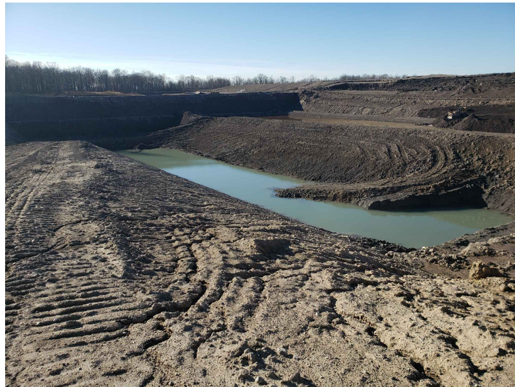
17 FORMER EAST SURFACE WATER POND - CELL 20-1 EXCAVATION Fig 4A
