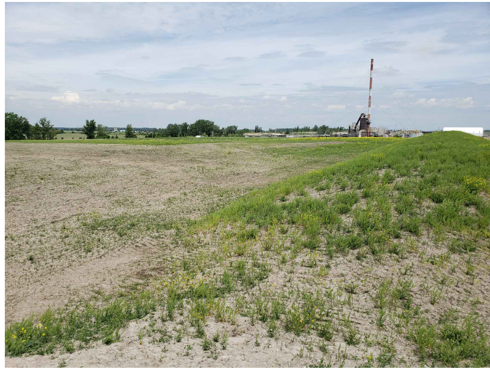
5 FINAL COVER - TOPSOIL PLACEMENT CELL 19-1 Fig 3A
