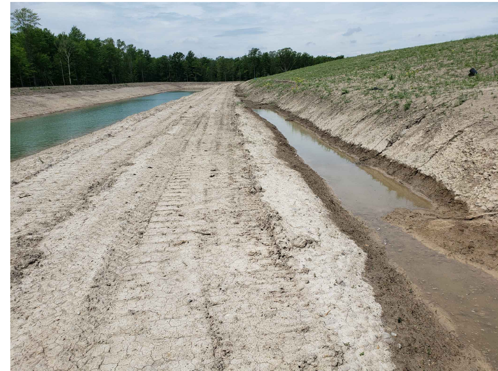
4 SOUTH ACCESS ROAD AND DITCH Fig 3A
