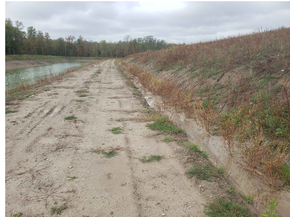
4 SOUTH ACCESS ROAD AND DITCH Fig 3A
