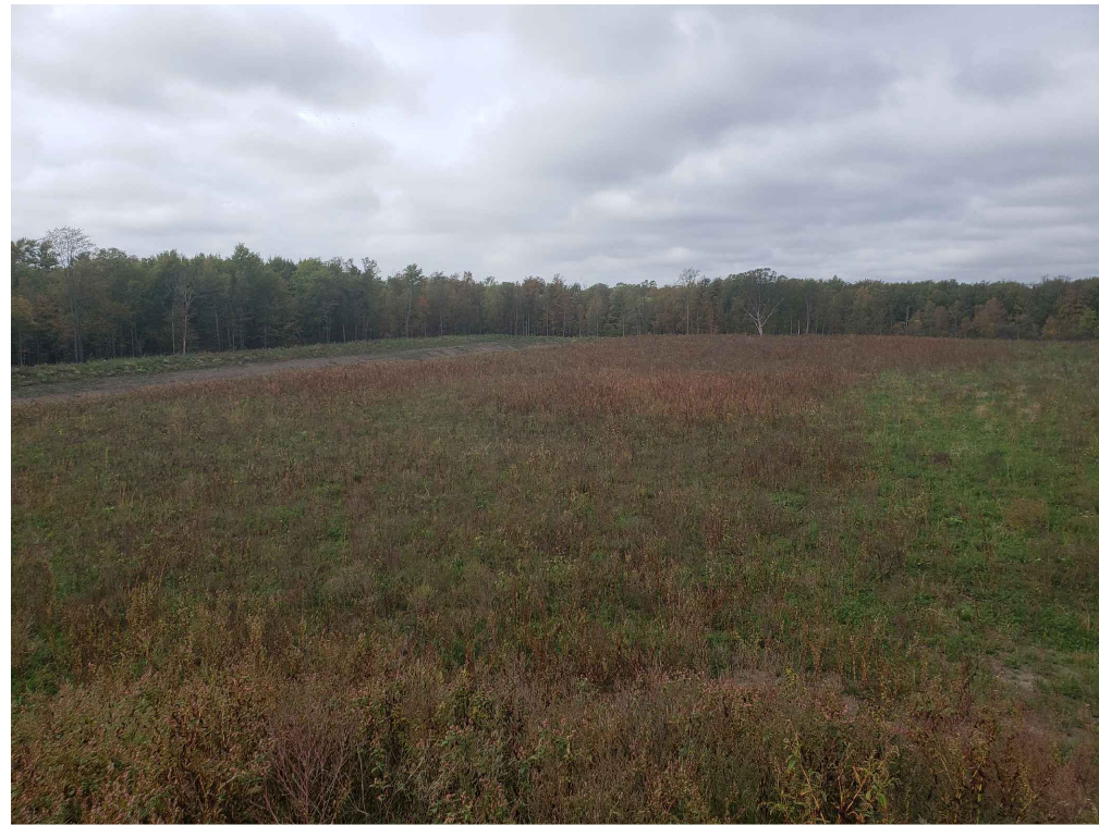
5 FINAL COVER - TOPSOIL PLACEMENT CELL 19-1 Fig 3A
