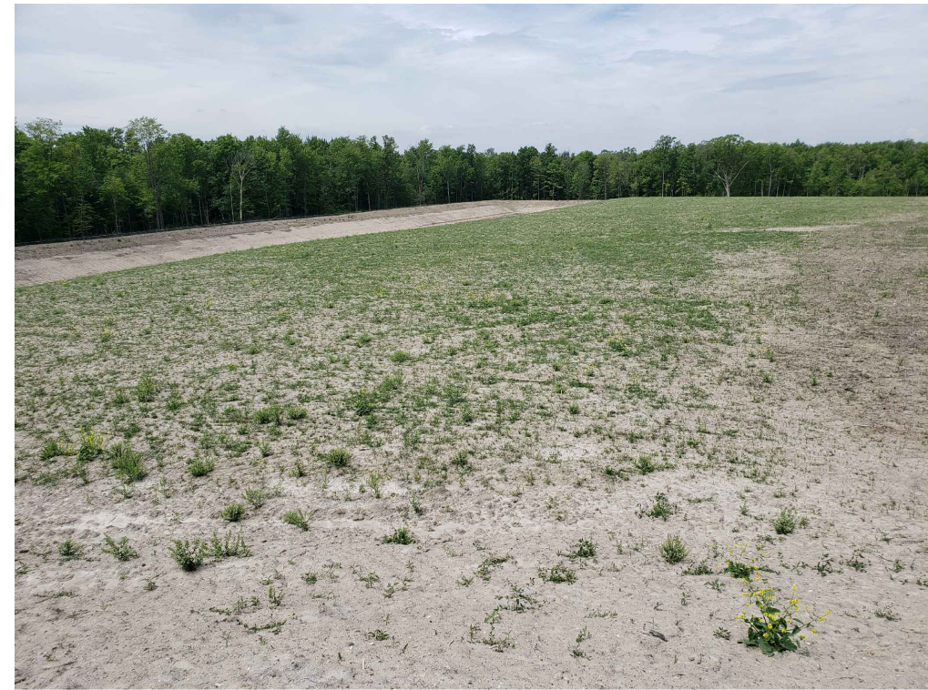
6 FINAL COVER - TOPSOIL PLACEMENT CELL 19-1 Fig 3A
