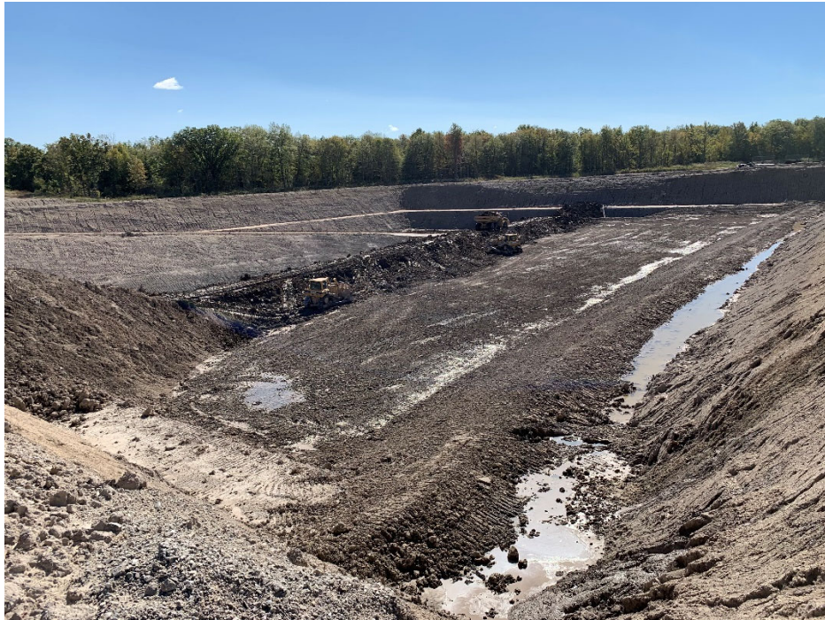
Photo 5- Completed buttness, looking southeast, September 30, 2021.
