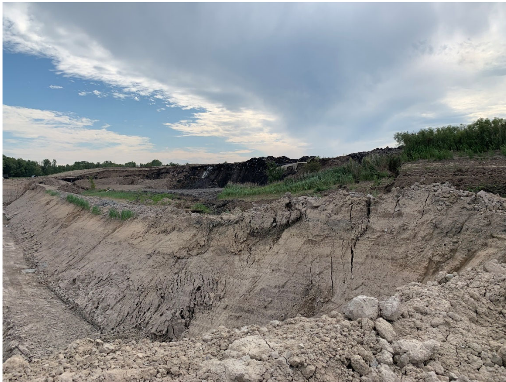
Photo 2- West side wall of Cell 20-1, looking south, August 18, 2021.
