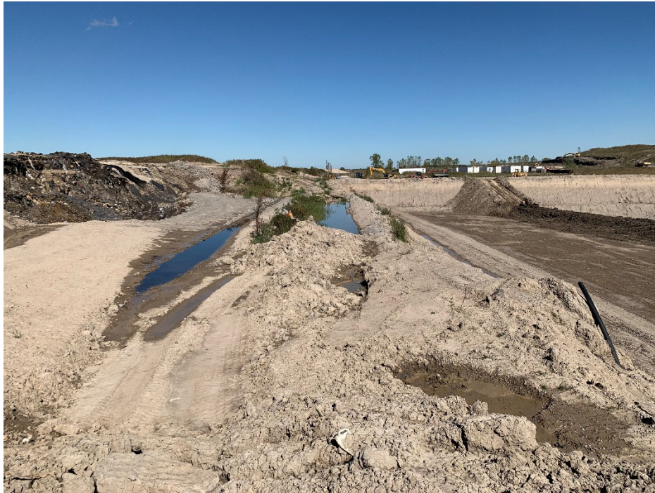
Photo 6- Completed buttness, looking north, September 30, 2021.
