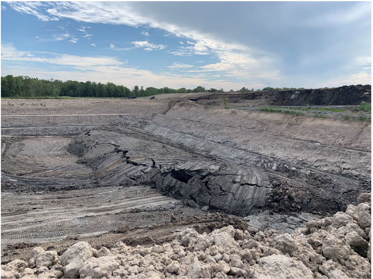
Photo 1- West Side wall of Cell 20-1, after slope movement, August 18, 2021.
