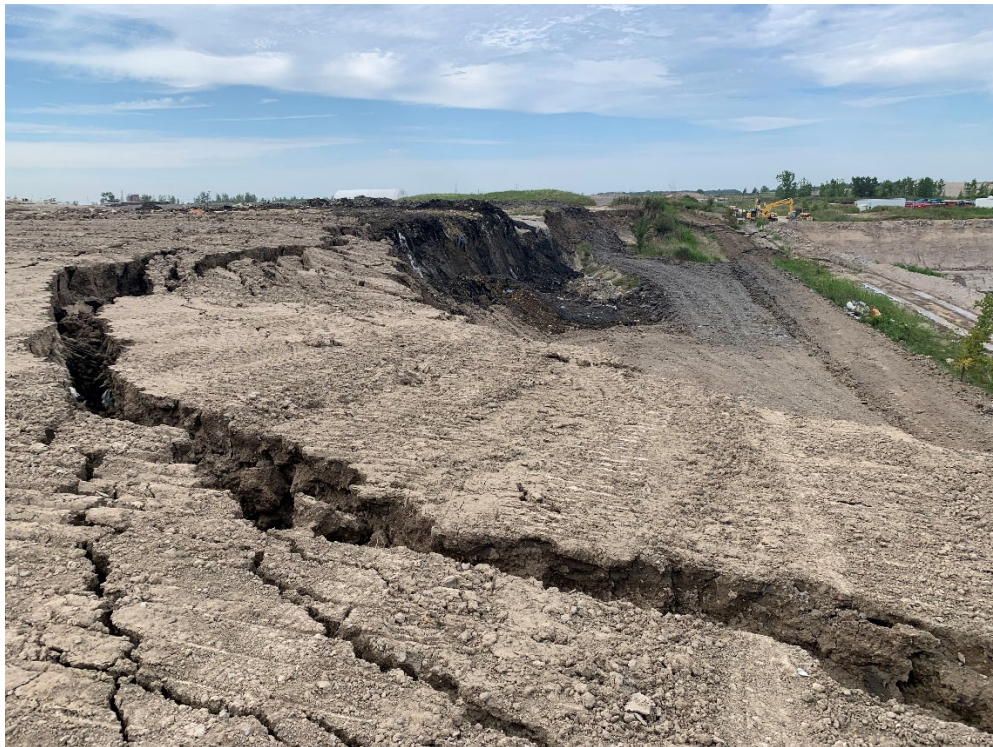
Photo 3- Top of Slide Area, looking north, August 18, 2021.
