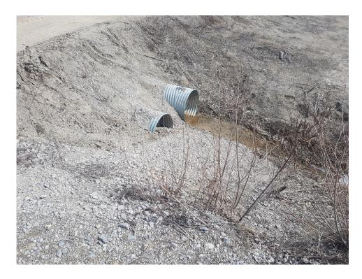
Photo 15 – Partially buried culvert at borrow area entrance
