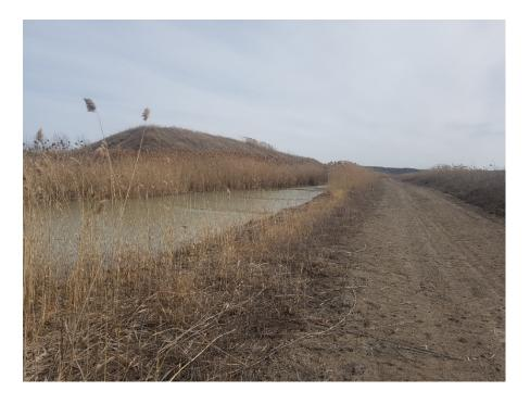
Photo 10 - High water levels in central portion of north perimeter ditch
