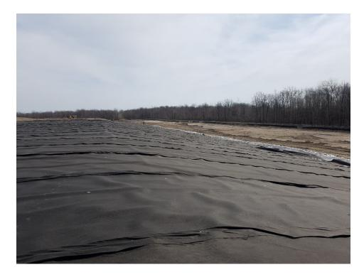
Photo 6 - Final landfill cover placement, Cell 19-1
