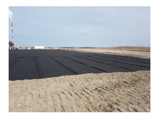
Photo 7 - Protective soil cover on Cell 19-1 final cover
