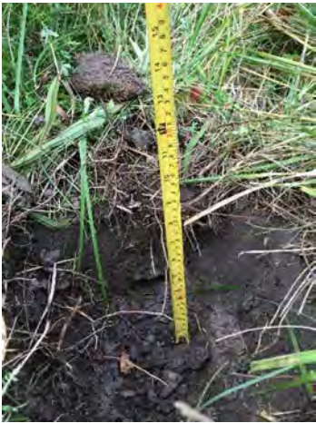
Photo 15: Installing ball-marker at S7
