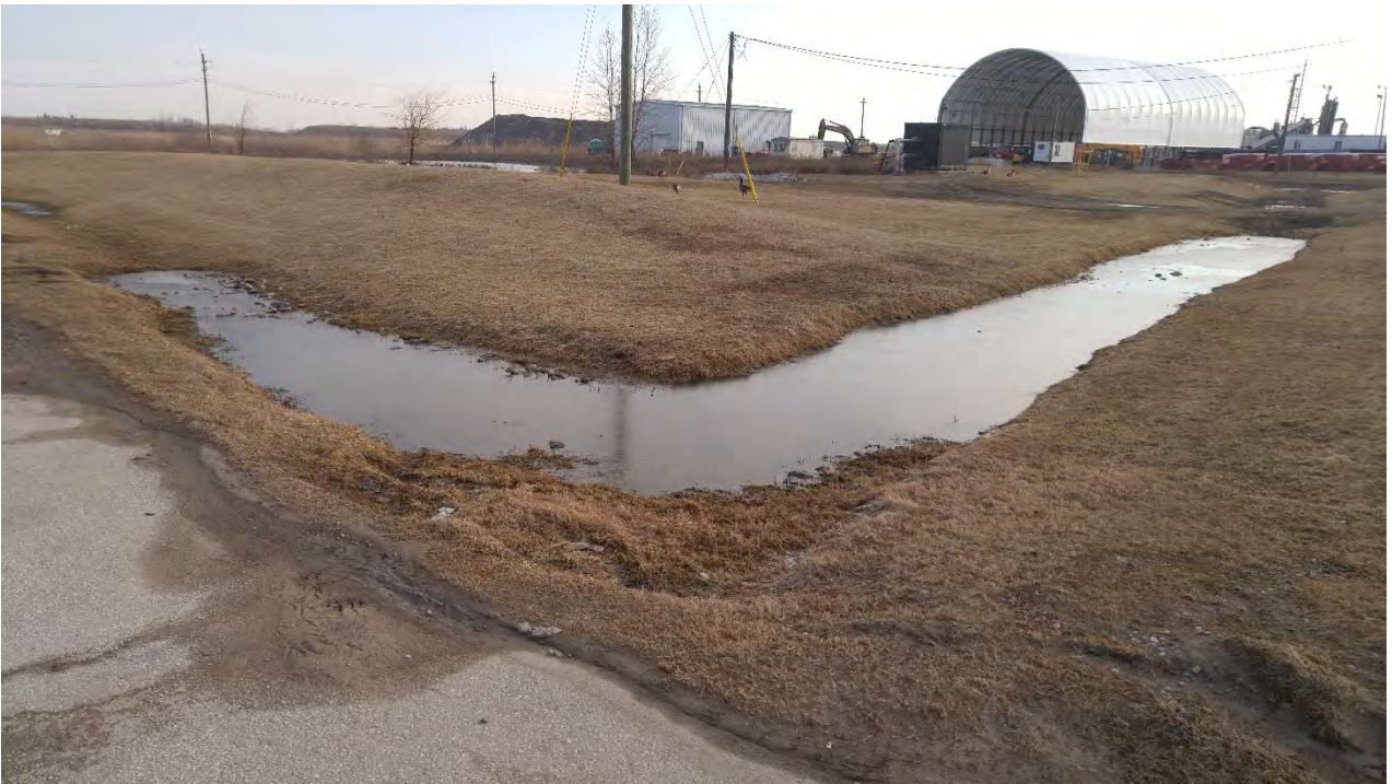
Photo 13 - North Process Water Pond ditch
