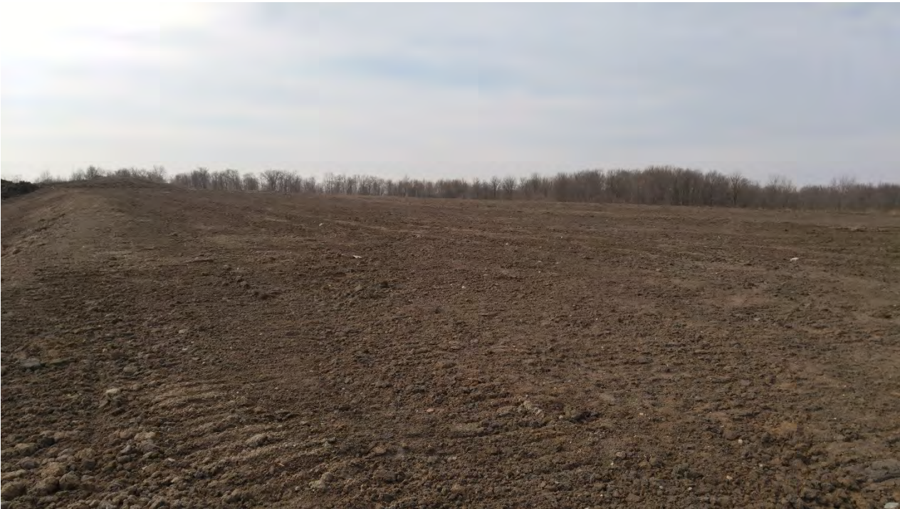
Photo 2 - Interim cap placement, Cell 19-1
