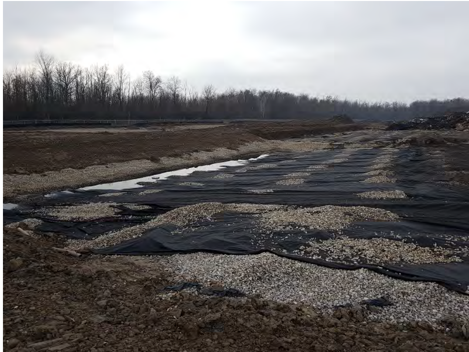
Photo 5 - Completed sub-cells, Cell 19-2
