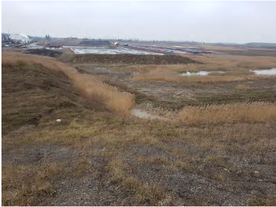
Photo 11 - Original Landfill Area, southeast ditch, sitting surface water
