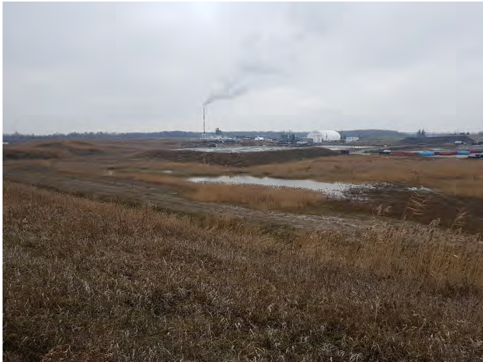
Photo 12 - Standing water in southeast corner of Original Landfill Area
