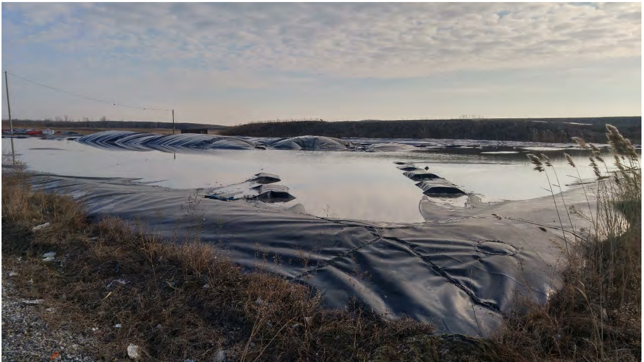
Photo 17 - East Leachate Reservoir
