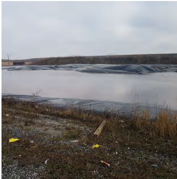
Photo 23 - New Leachate Reservoir
