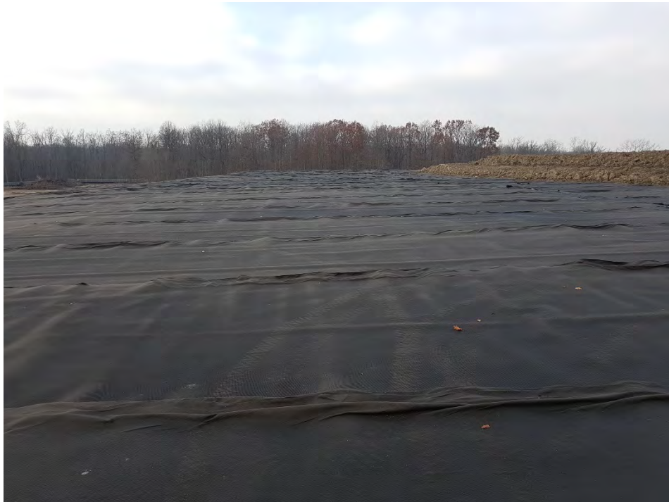
Photo 6 - Final landfill cover placement, Cell 19-1
