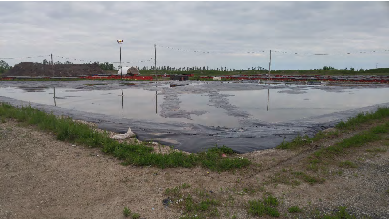
Photo 16 - South Leachate Reservoir
