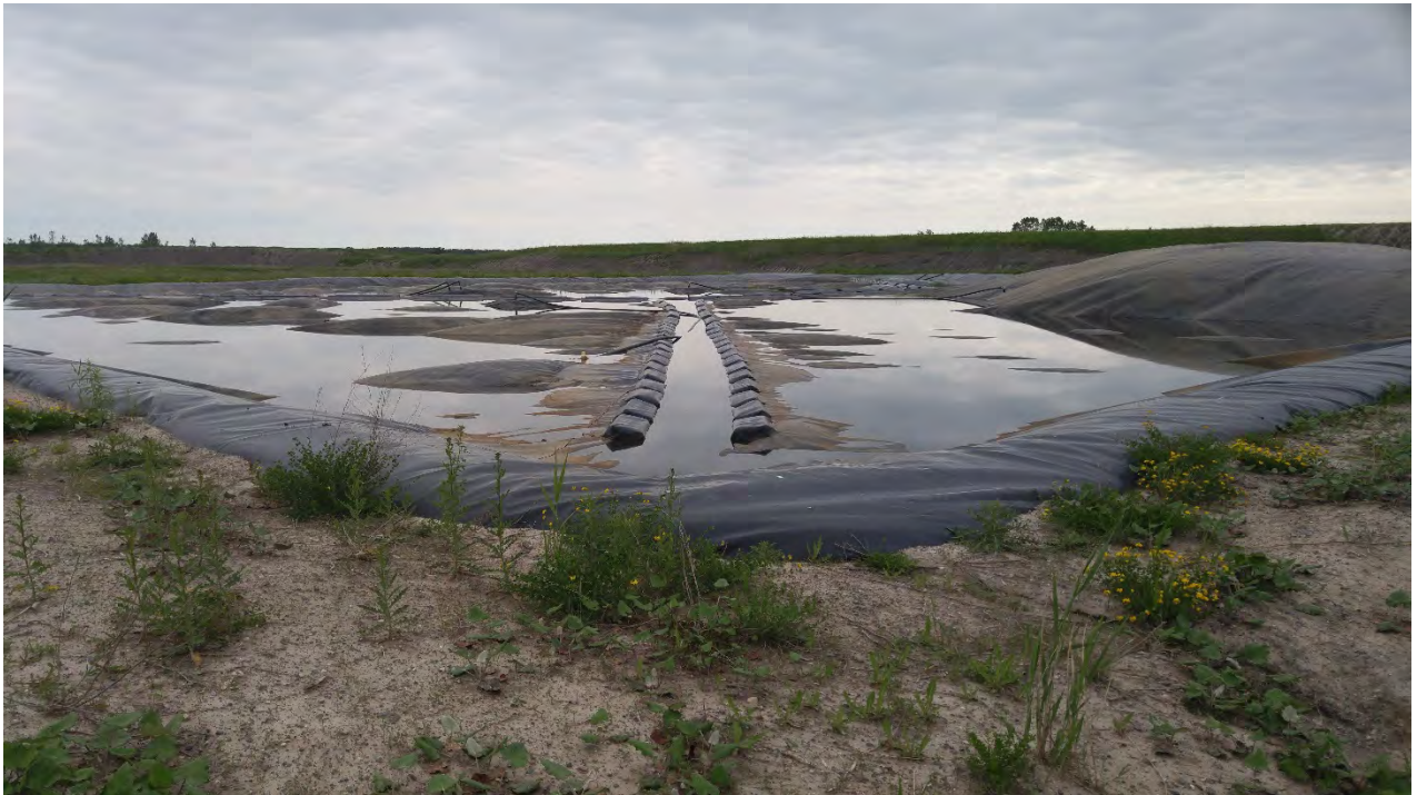
Photo 18 - New Leachate Reservoir
