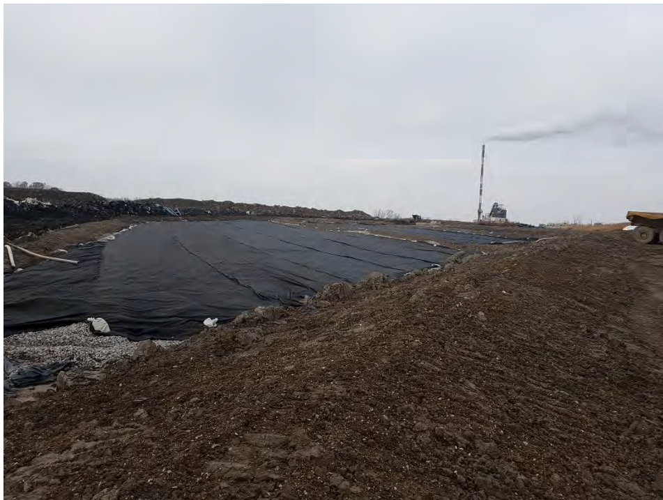
Photo 2 – Completed sub-cells, Cell 19-2
