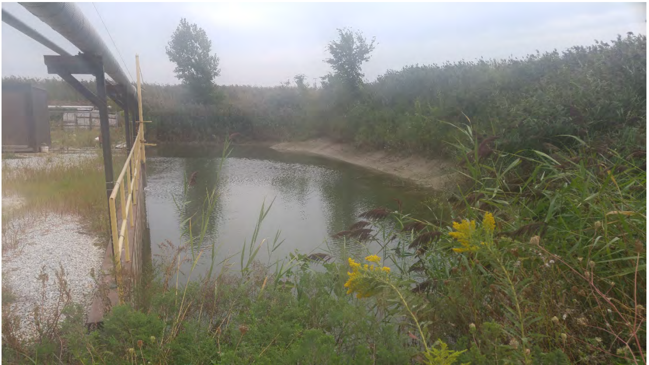
Photo 15 - South Process Water Pond
