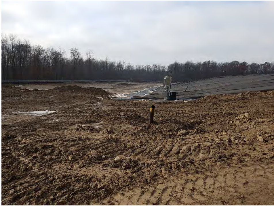
Photo 13 – Completed south ditch remediation
