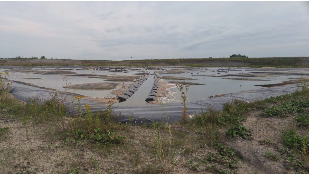
Photo 18 - New Leachate Reservoir
