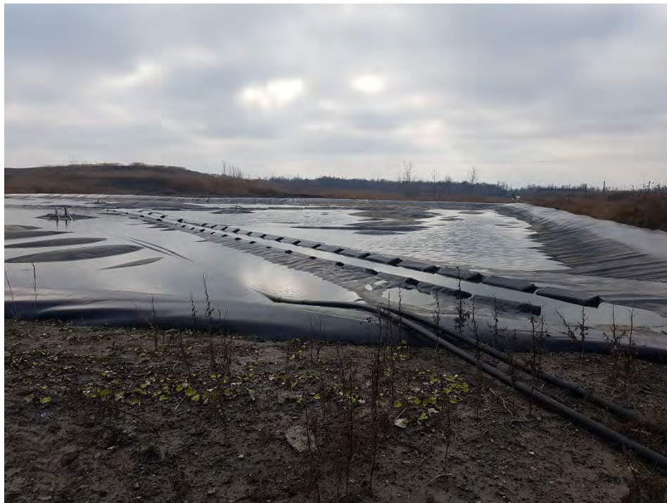
Photo 22 - East Leachate Reservoir
