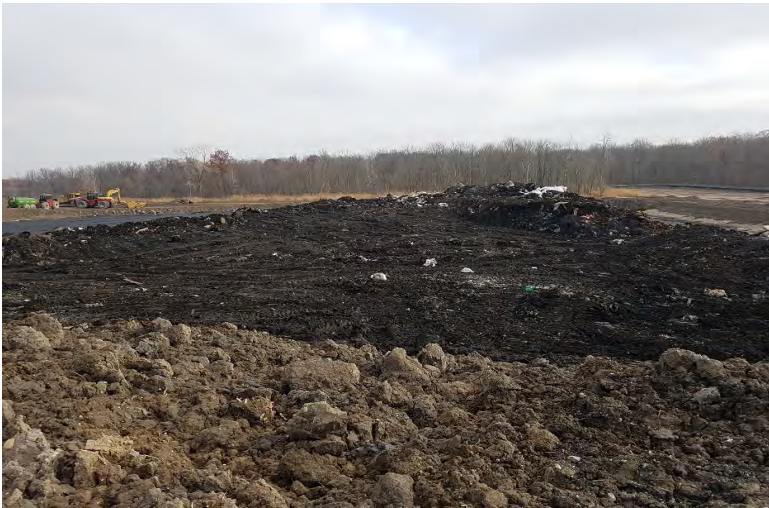
Photo 1 - Active landfilling cell, Cell 19-2
