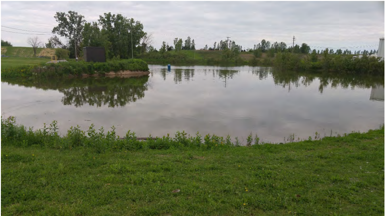
Photo 14 - North Process Water Pond
