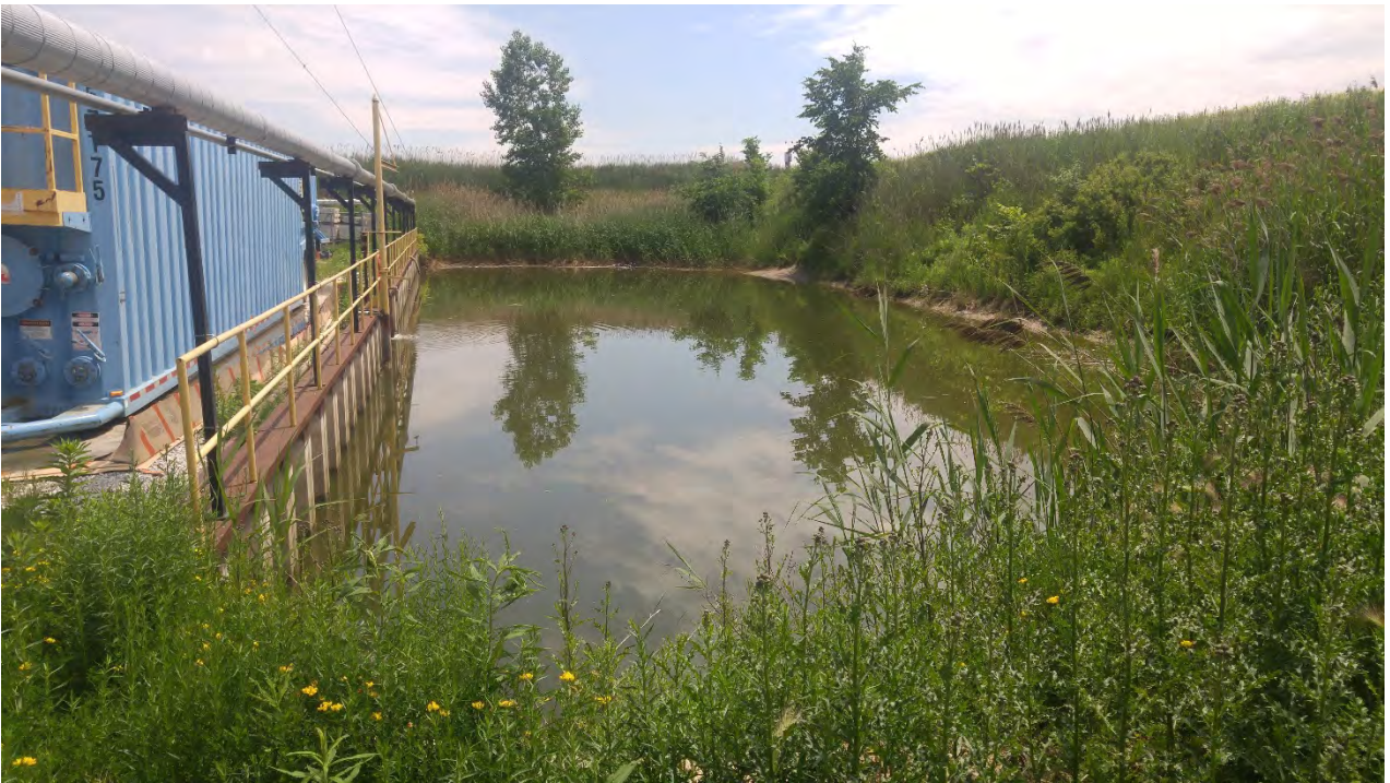
Photo 15 - South Process Water Pond
