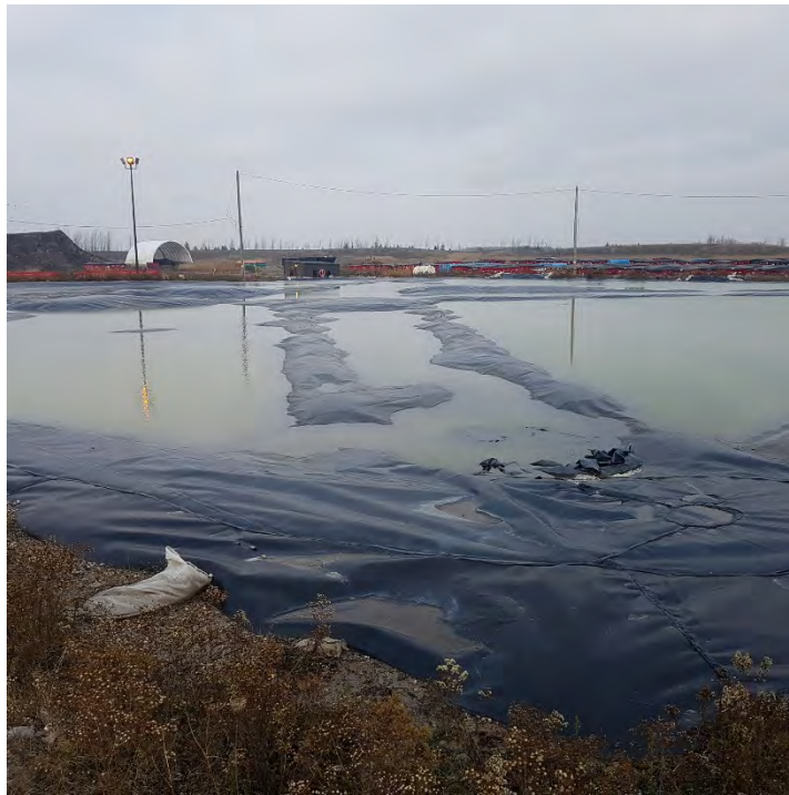
Photo 21 - South Leachate Reservoir
