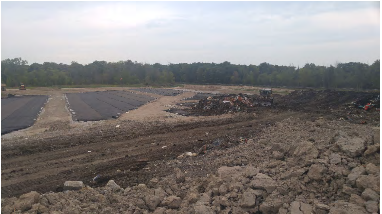
Photo 1 - Active landfilling cell and cell construction, Cell 19-2
