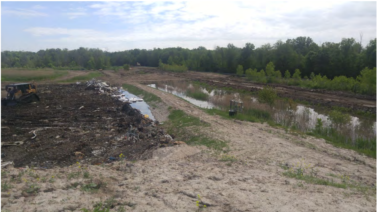
Photo 9 - South ditch remediation
