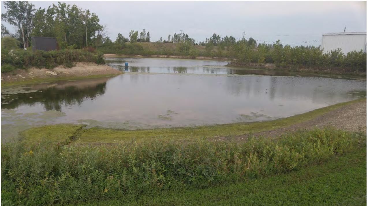
Photo 14 - North Process Water Pond
