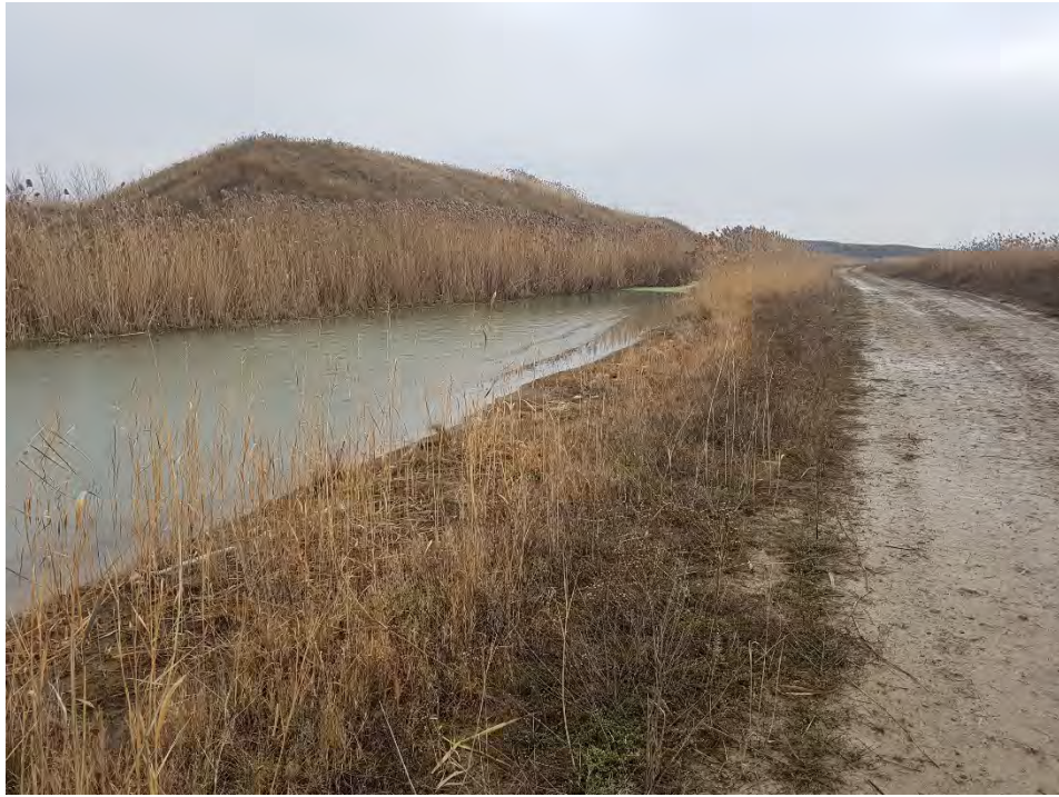
Photo 9 - High water levels in central portion of north perimeter ditch
