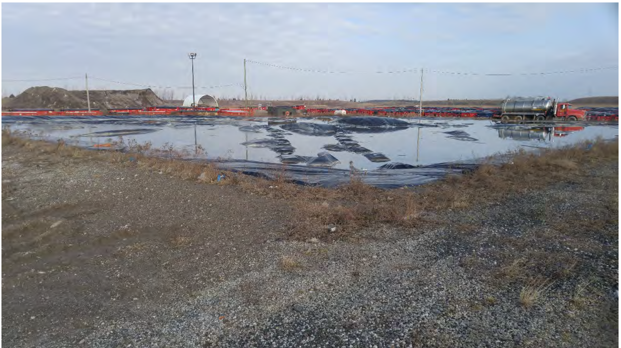
Photo 16 - South Leachate Reservoir
