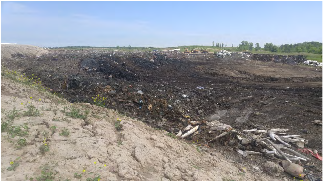
Photo 1 - Active landfilling cell, Cell 19-2A
