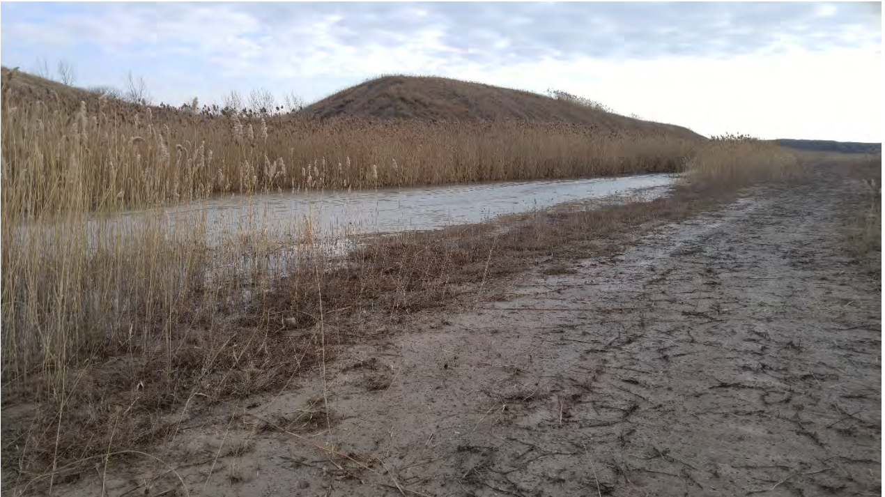
Photo 5 - High water levels in central portion of north perimeter ditch, ice cover
