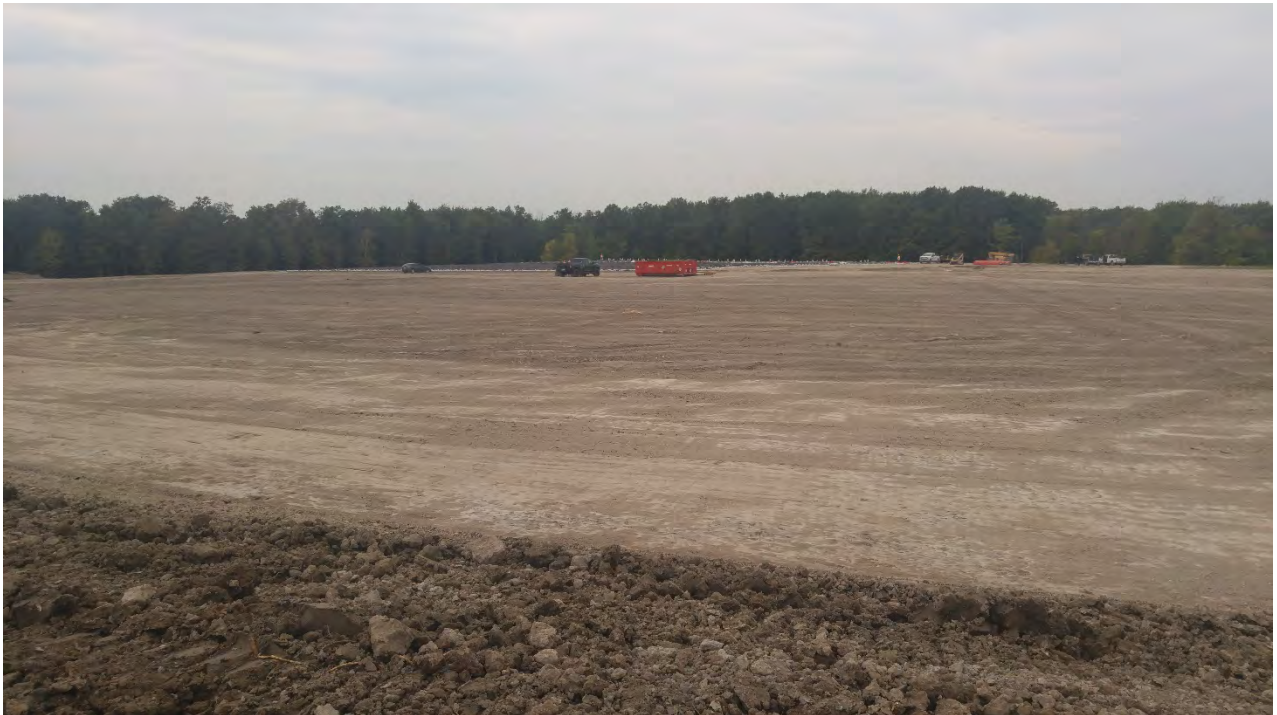
Photo 2 - Interim and final cap placement, Cell 19-1
