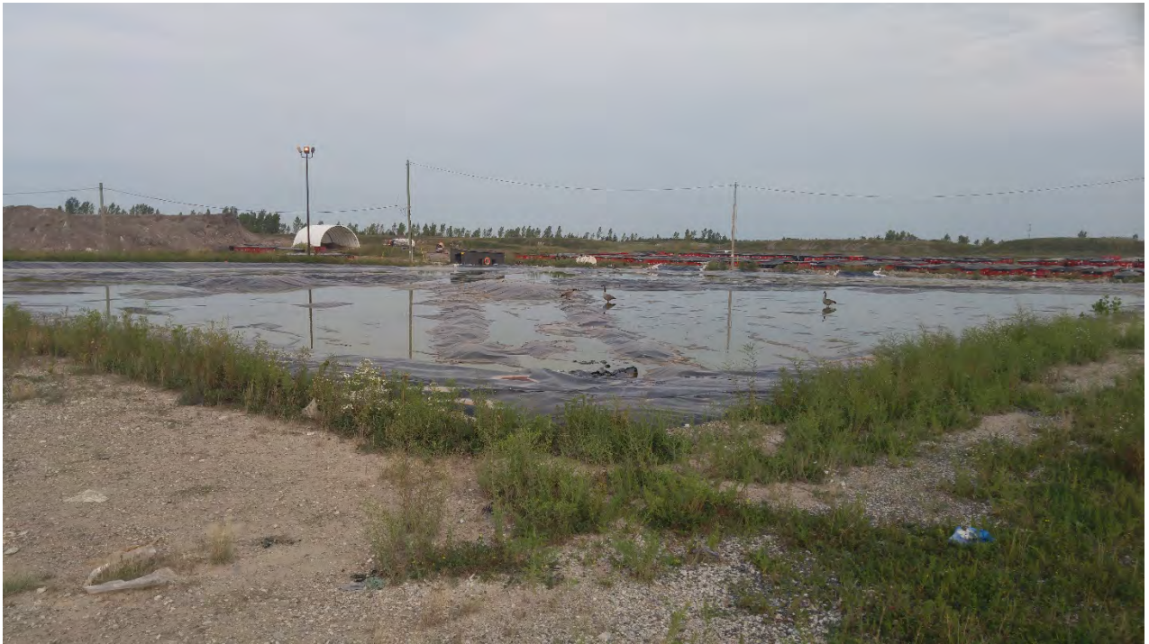
Photo 16 - South Leachate Reservoir
