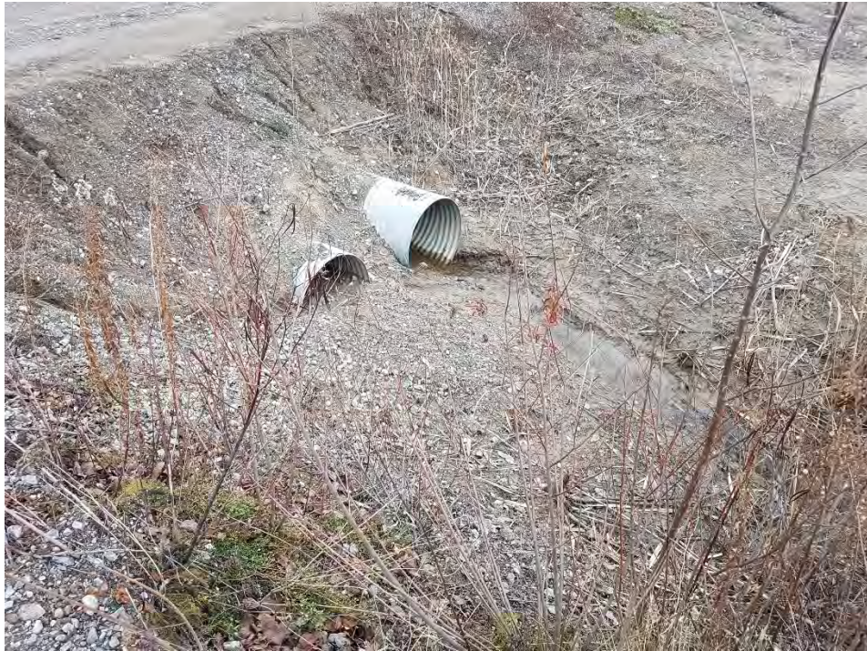
Photo 15 – Partially buried culver at barrow area entrance
