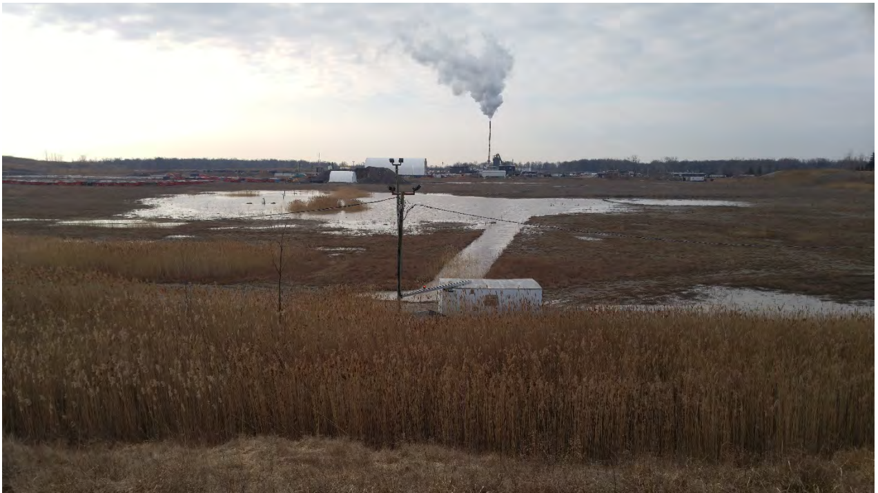
Photo 3 - Standing water in northwest corner of Site
