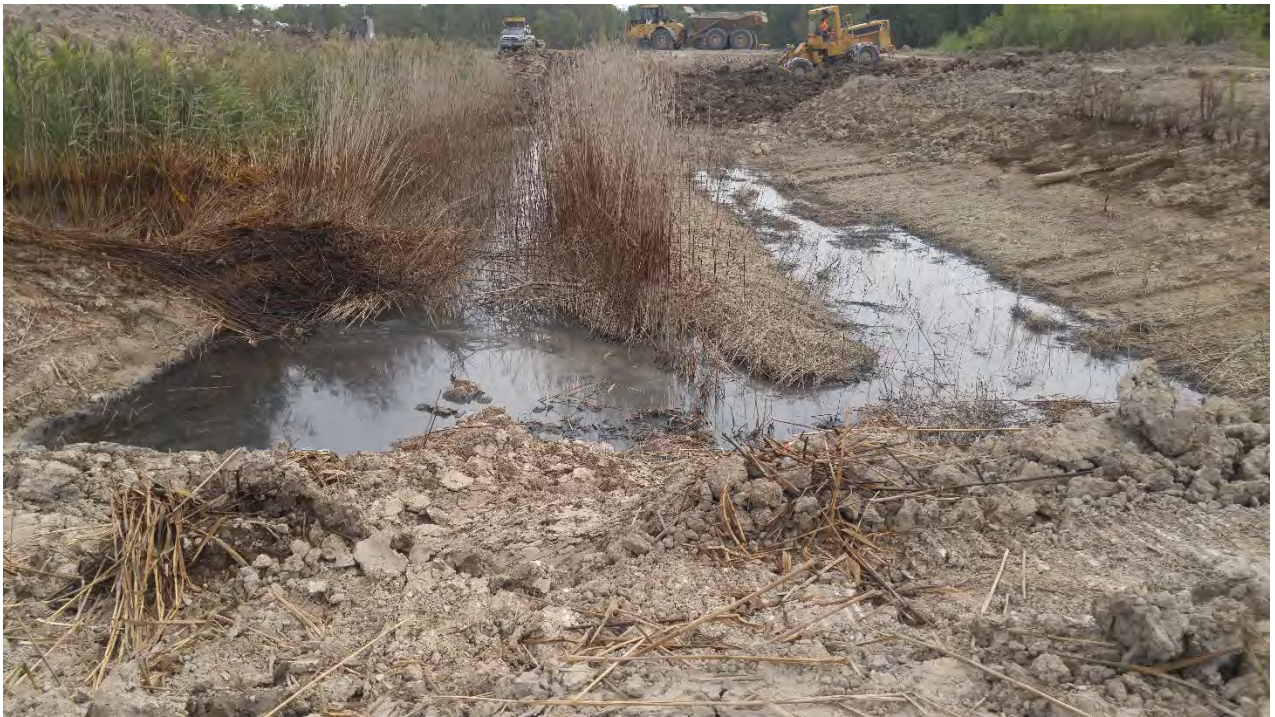
Photo 9 - South ditch remediation
