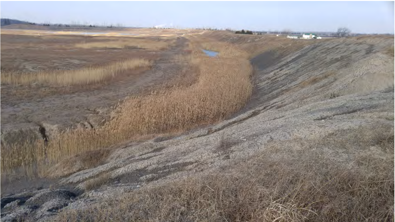
Photo 6 - North ditch, surface water blockage
