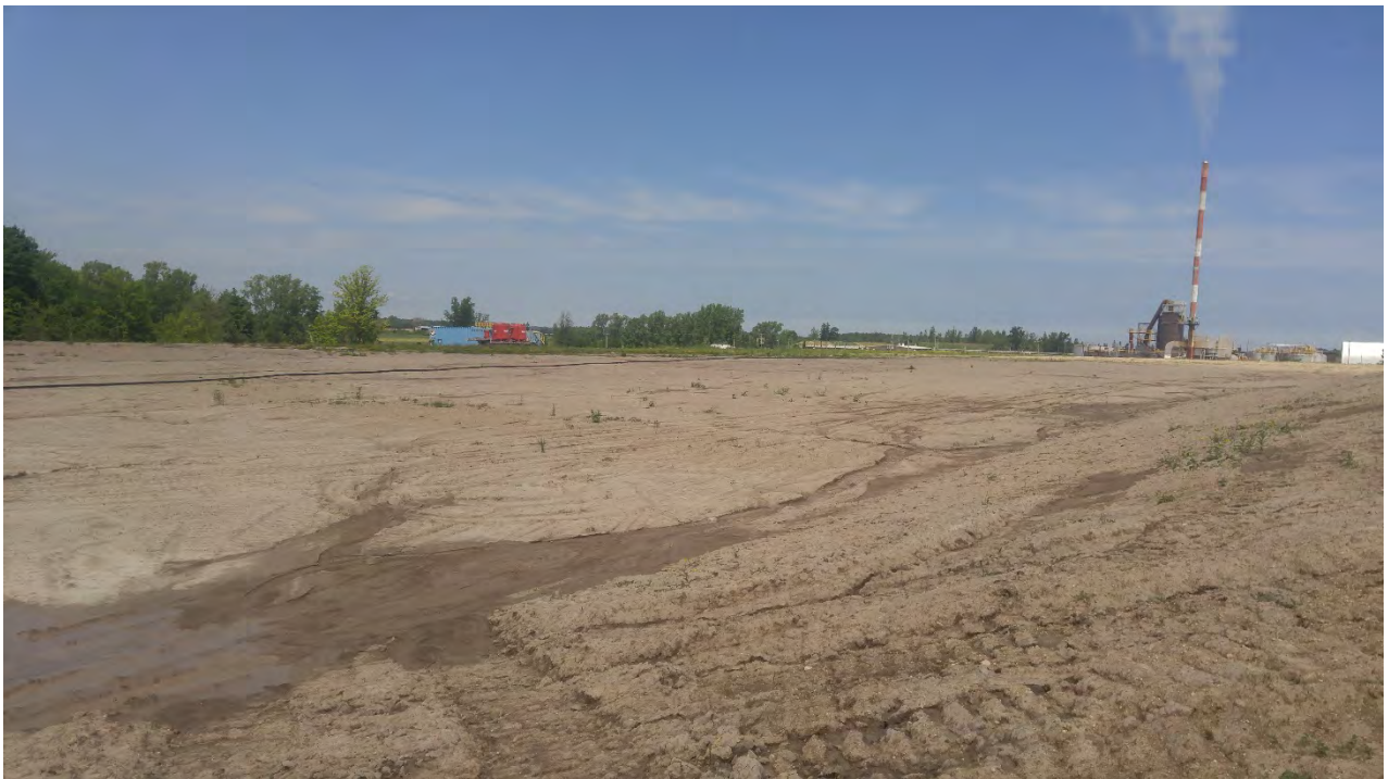
Photo 2 - Interim cap placement, Cell 19-1
