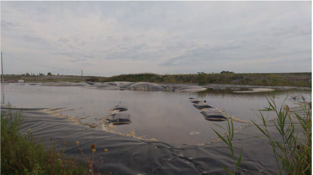
Photo 17 - East Leachate Reservoir
