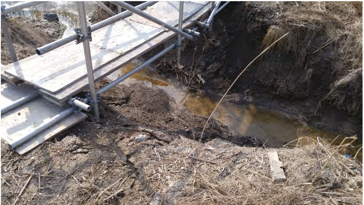
Photo 9 - South ditch, surface water blockage removed
