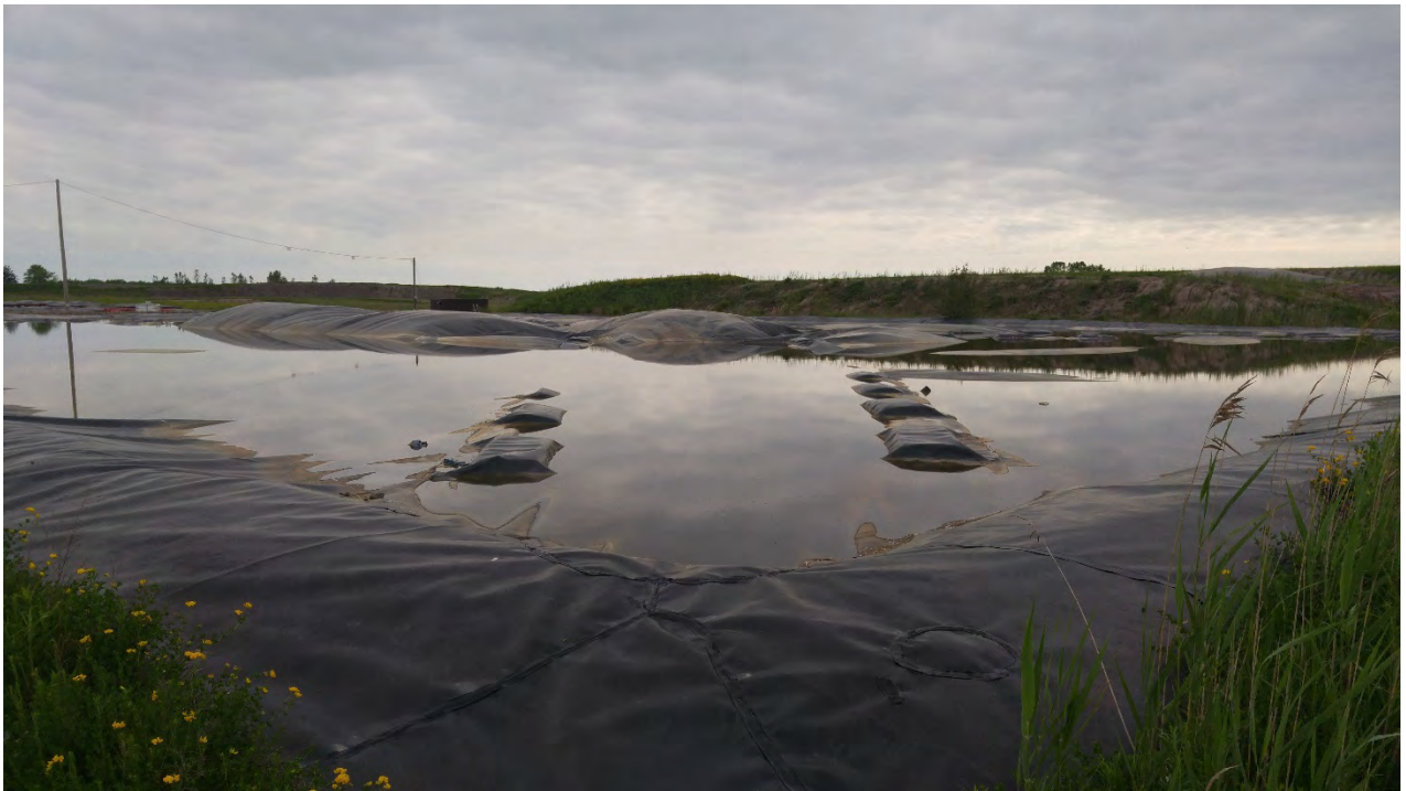
Photo 17 - East Leachate Reservoir
