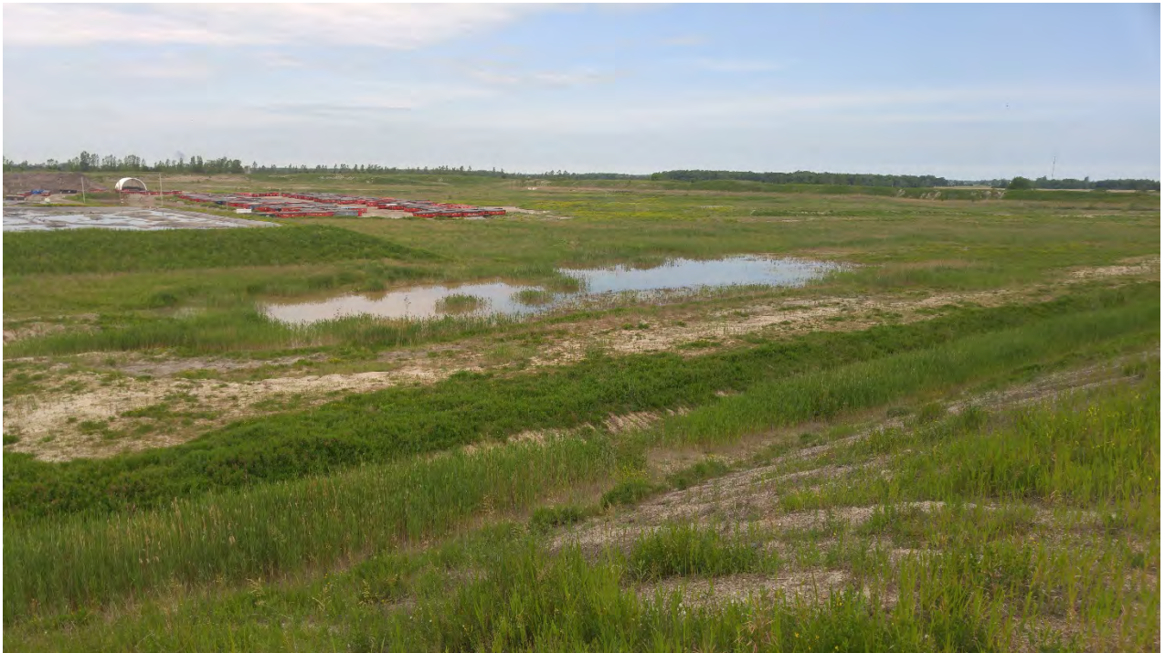
Photo 8 - Standing water in southeast corner of north landfill area
