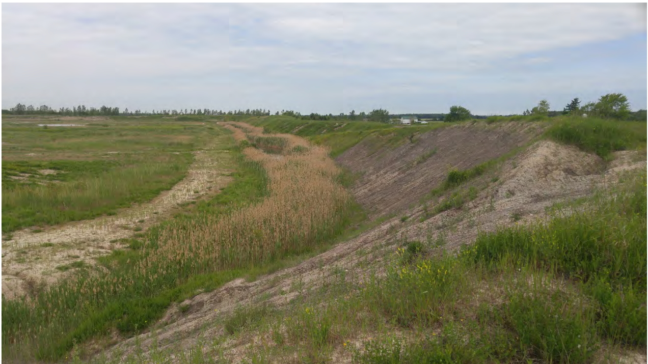
Photo 6 - North ditch, surface water blockage
