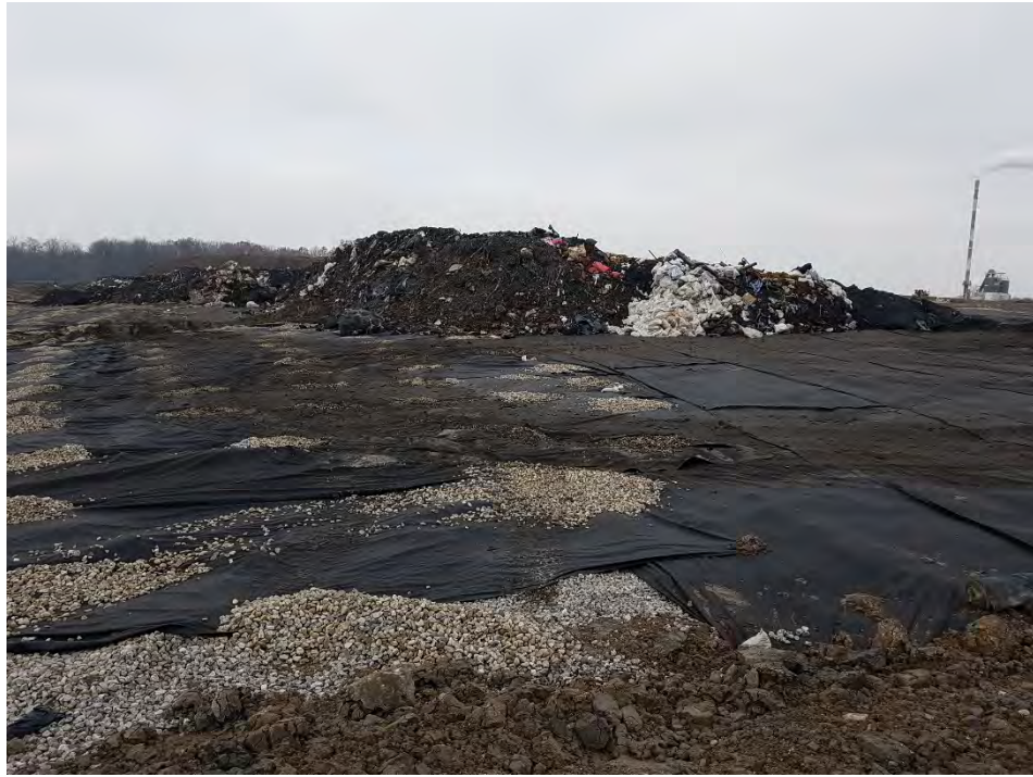
Photo 3 - Completed sub-cells, Cell 19-2
