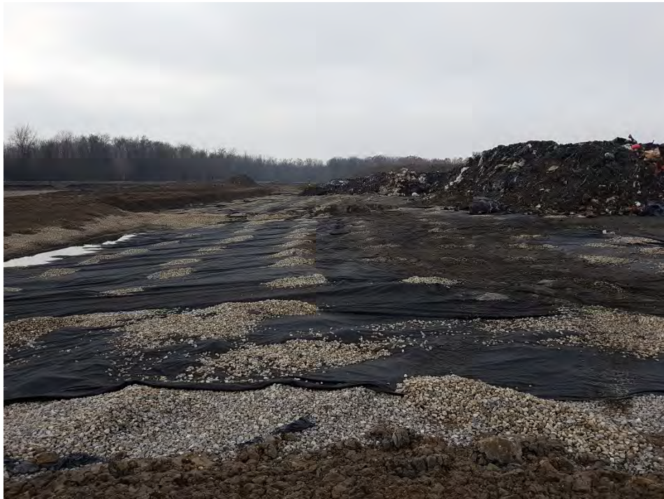
Photo 4 - Completed sub-cells, Cell 19-2
