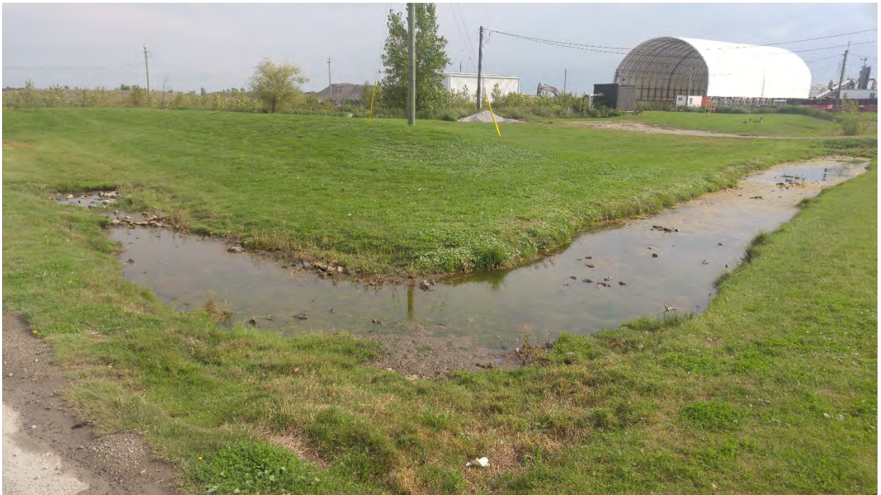
Photo 13 - North Process Water Pond ditch
