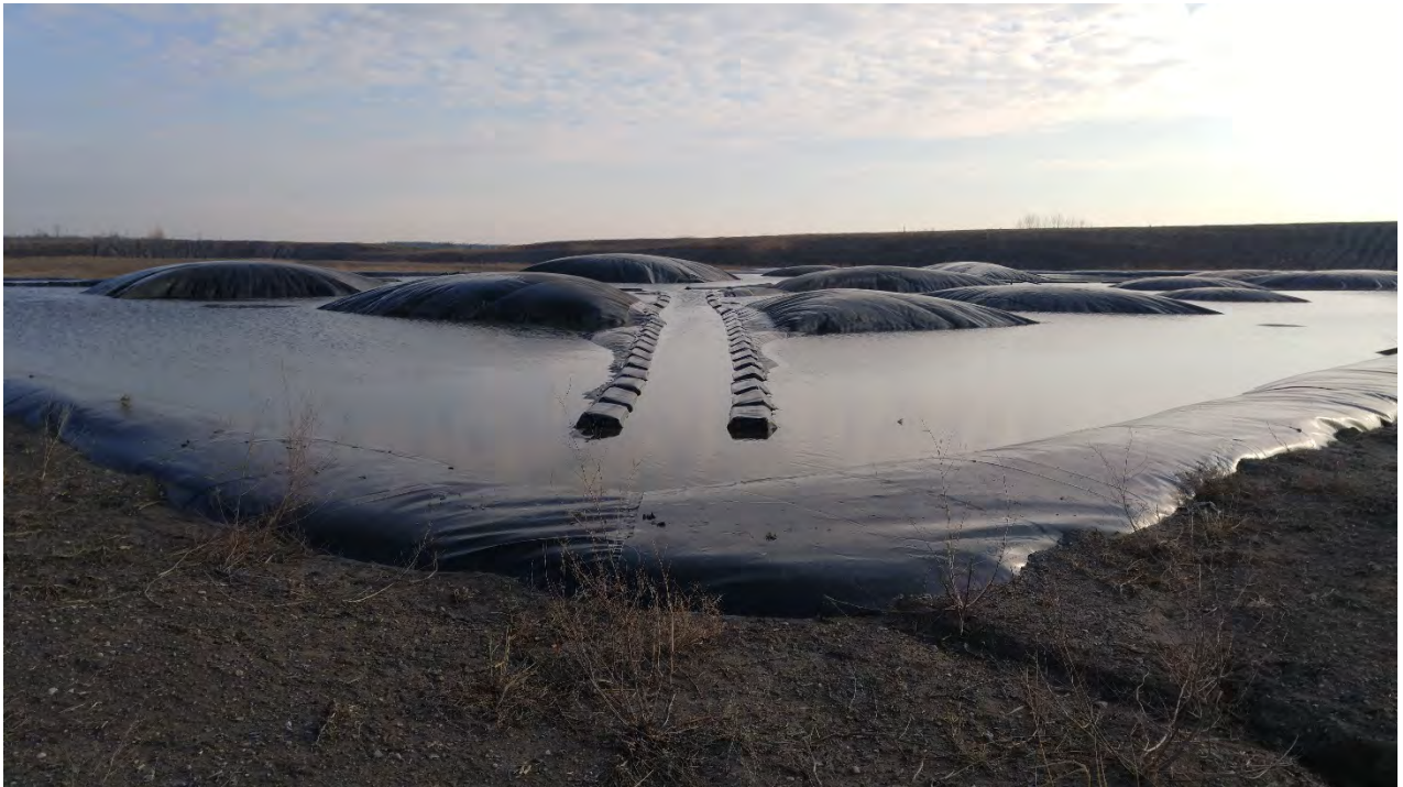
Photo 18 - New Leachate Reservoir
