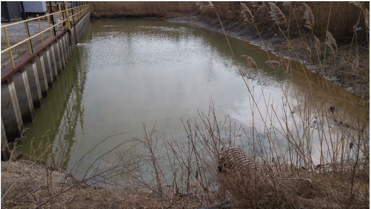
Photo 15 - South Process Water Pond
