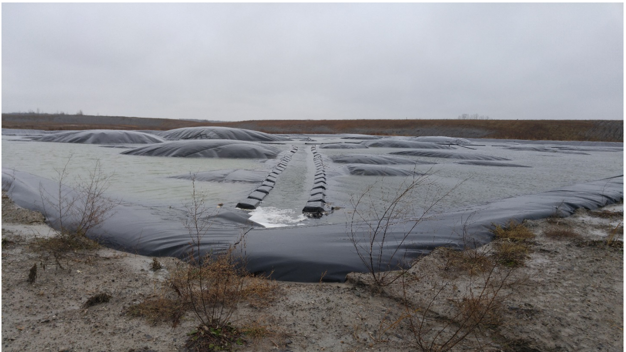
Photo 18 - New Leachate Reservoir
