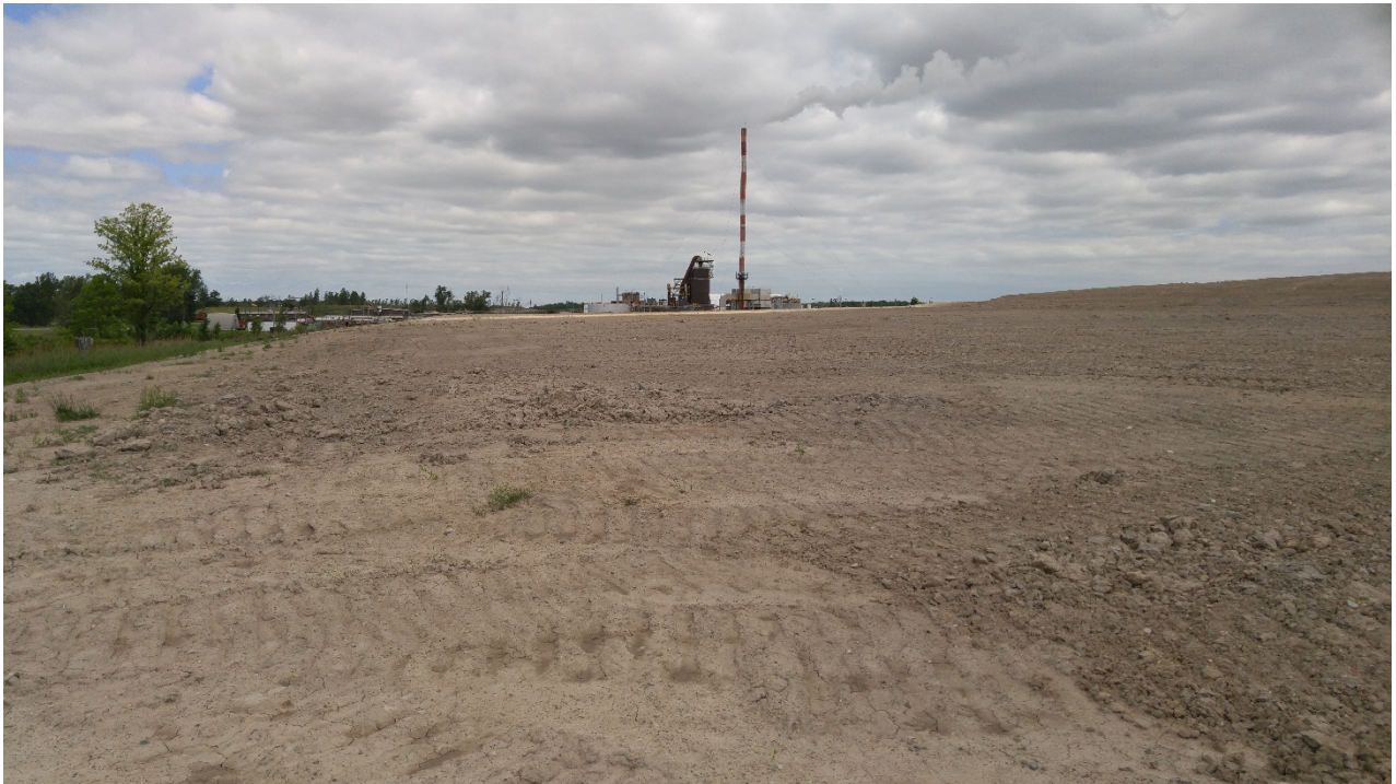
Photo 2 - Interim cap placement, Cells 19-1-1 and 19-1-2
