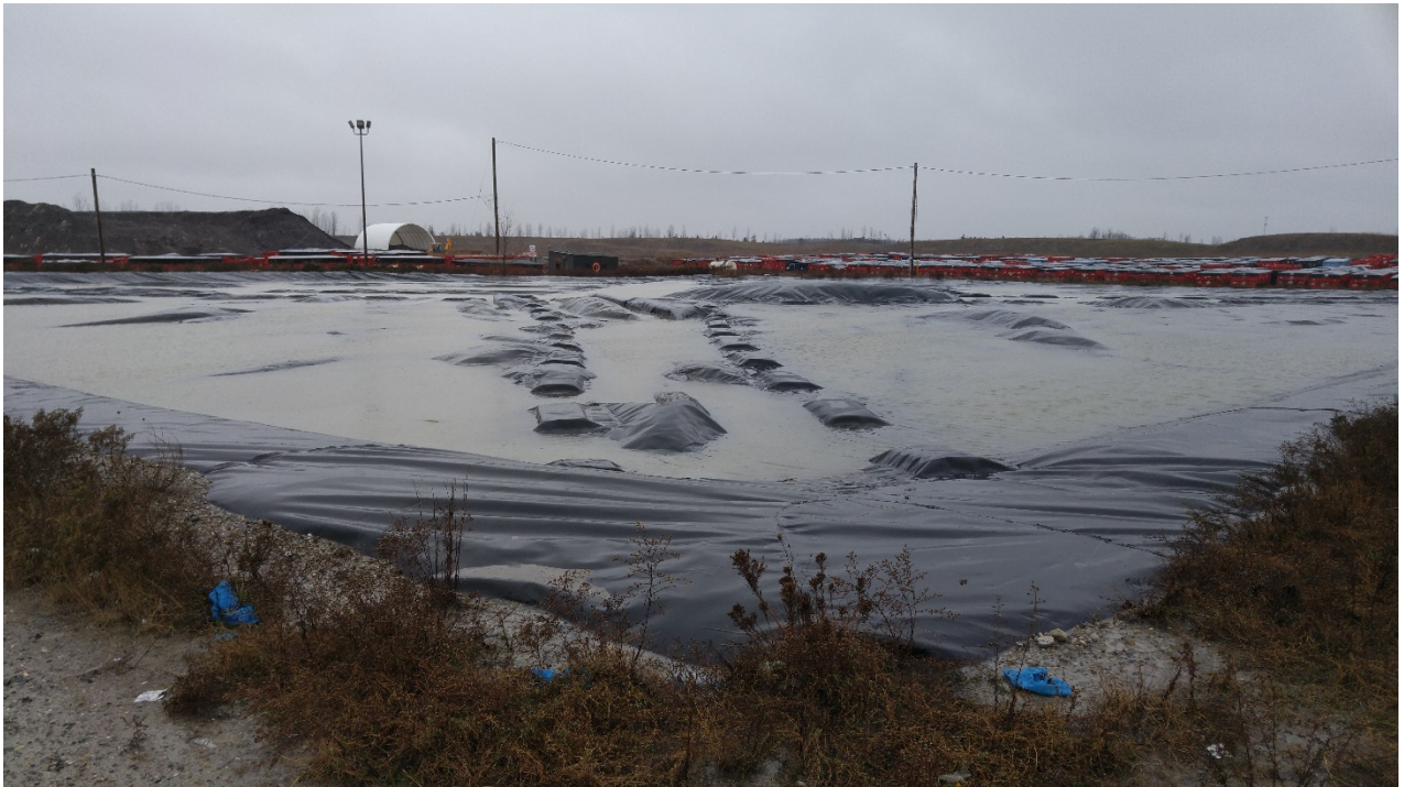
Photo 16 - South Leachate Reservoir
