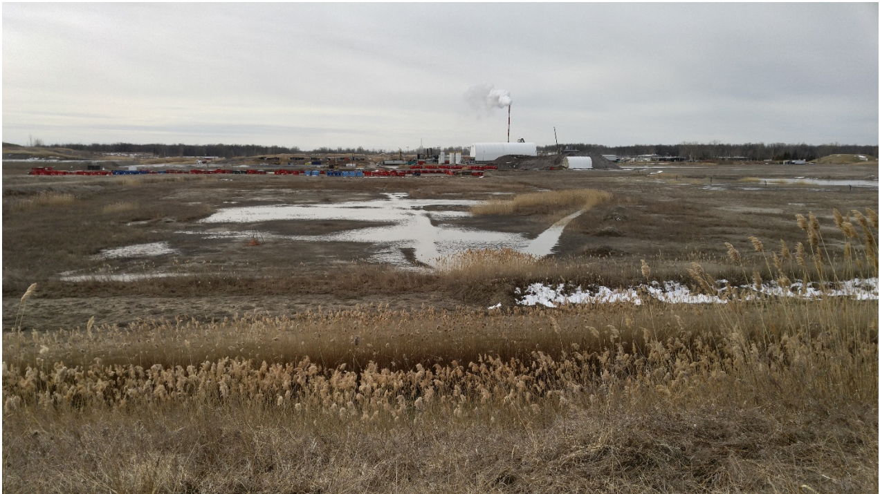
Photo 4 - Ponding in northern, central portion of Site
