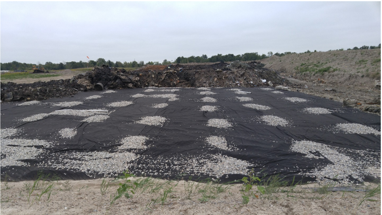
Photo 1 - Active landfilling cell (northern portion of Cell 19-1-3)
