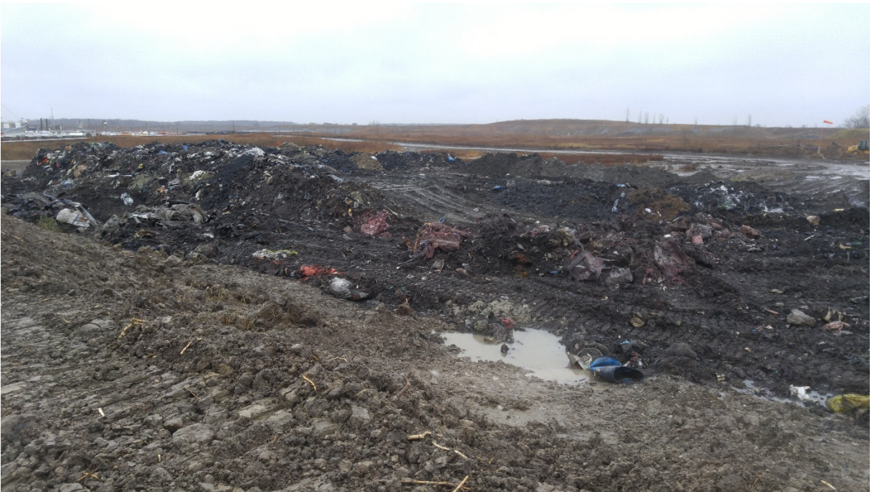
Photo 1 - Active landfilling cell (northern portion of Cell 19-1-3)
