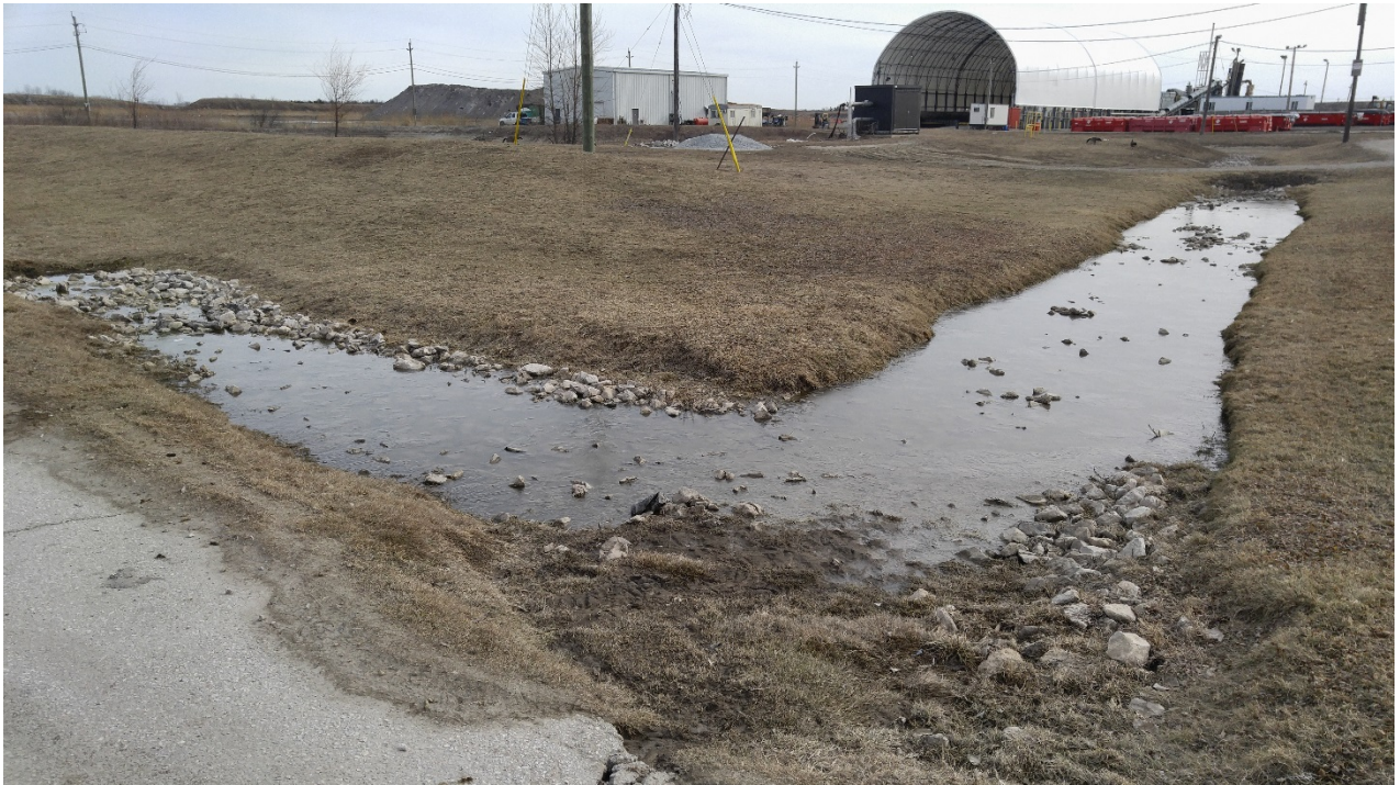
Photo 12 - North Process Water Pond ditch
