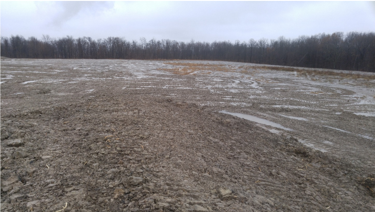
Photo 2 - Interim cap placement, Cells 19-1-1 and 19-1-2
