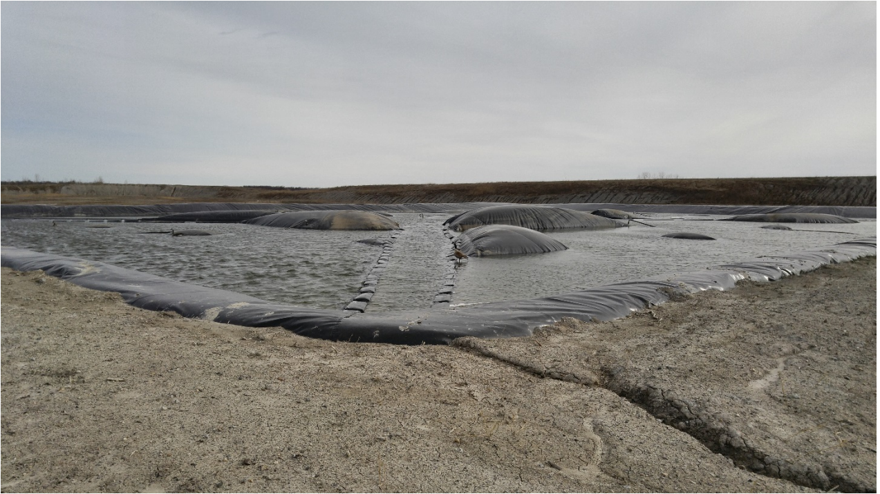
Photo 16 - New Leachate Reservoir
