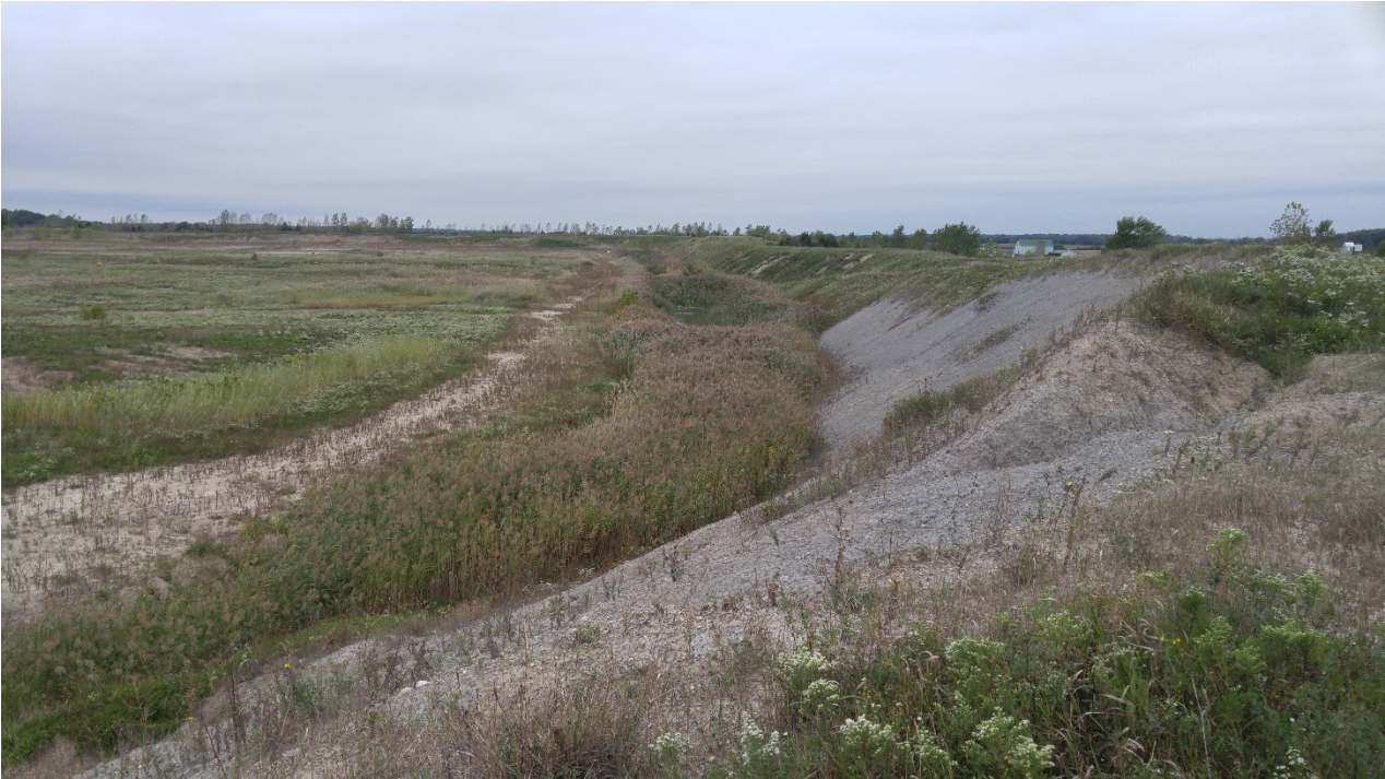
Photo 6 - North ditch, surface water blockage
