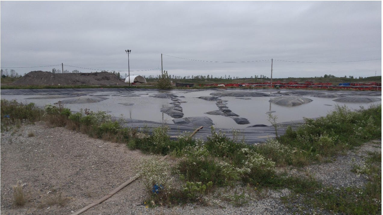
Photo 15 - South Leachate Reservoir
