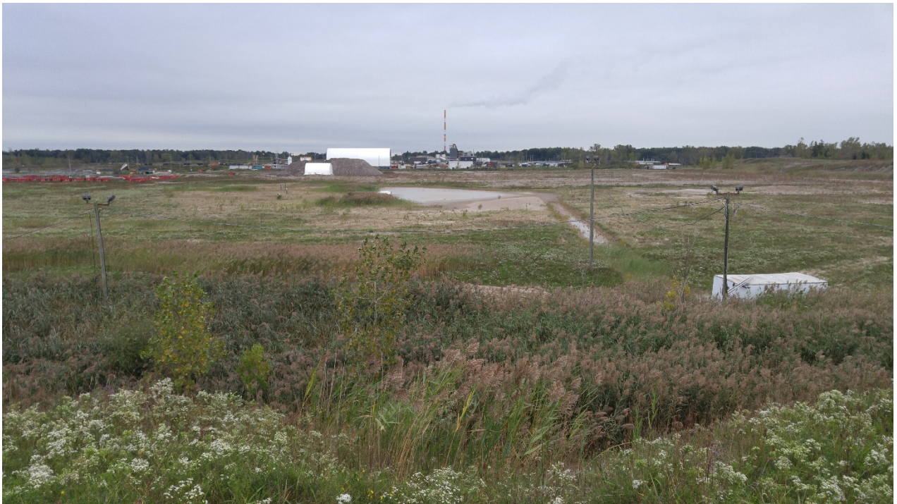
Photo 3 - Northwest corner of Site
