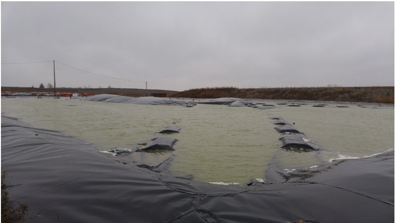
Photo 17 - East Leachate Reservoir
