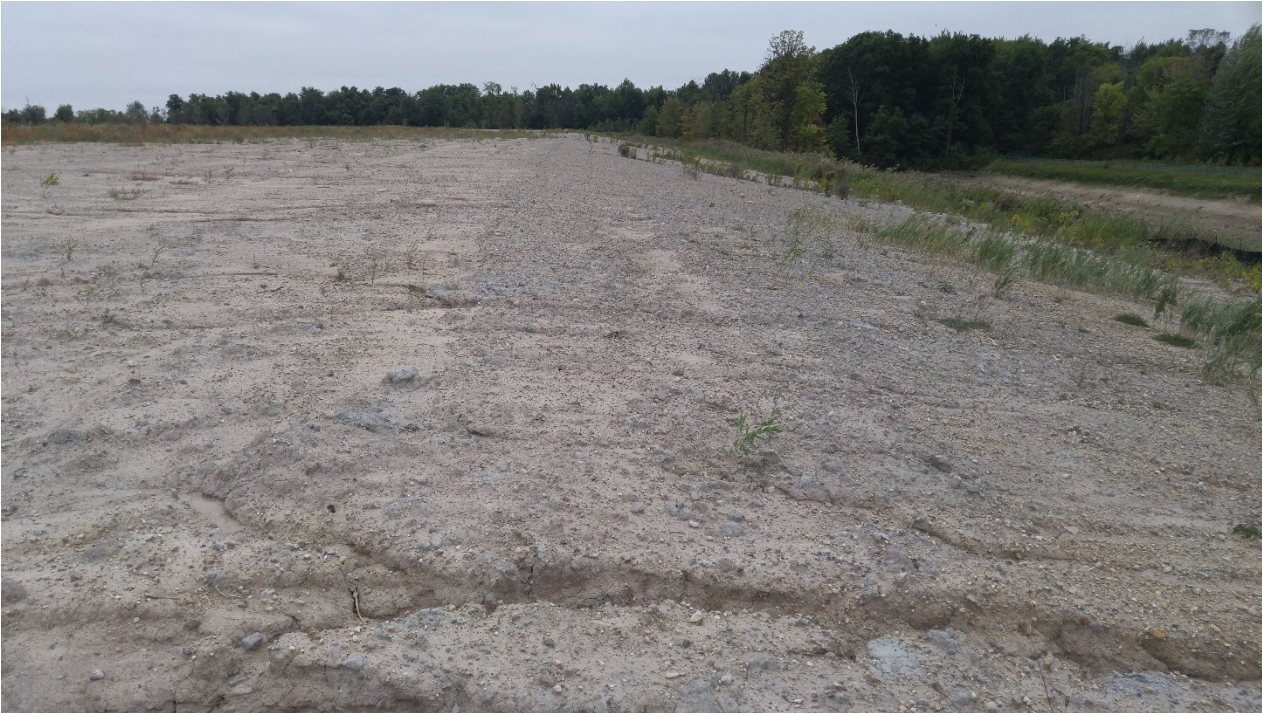
Photo 2 - Interim cap placement, Cells 19-1-1 and 19-1-2
