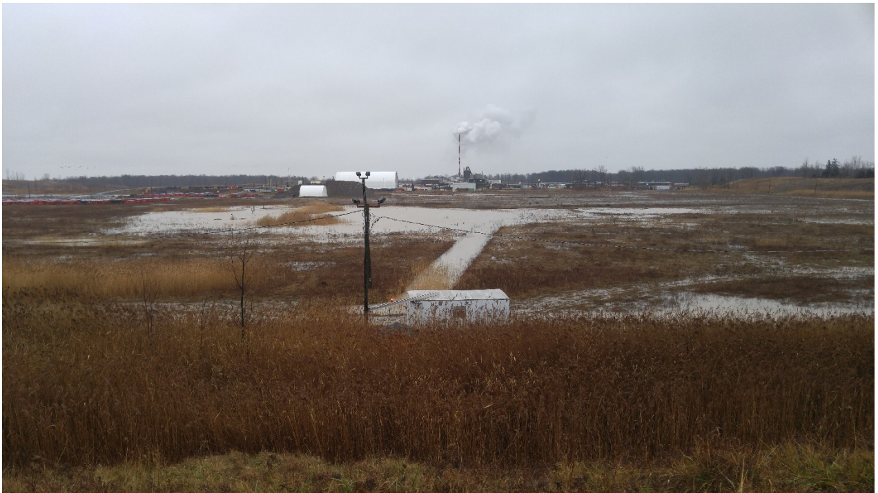
Photo 3 - Standing water in northwest corner of Site
