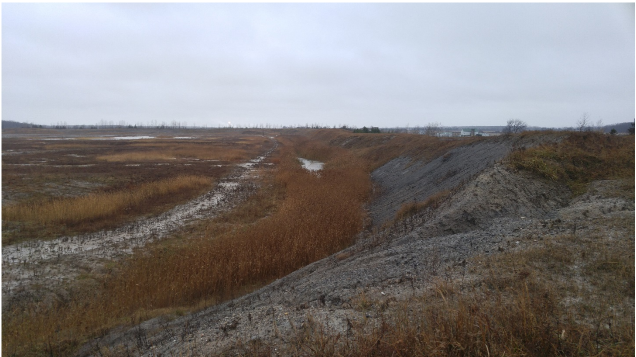
Photo 6 - North ditch, surface water blockage
