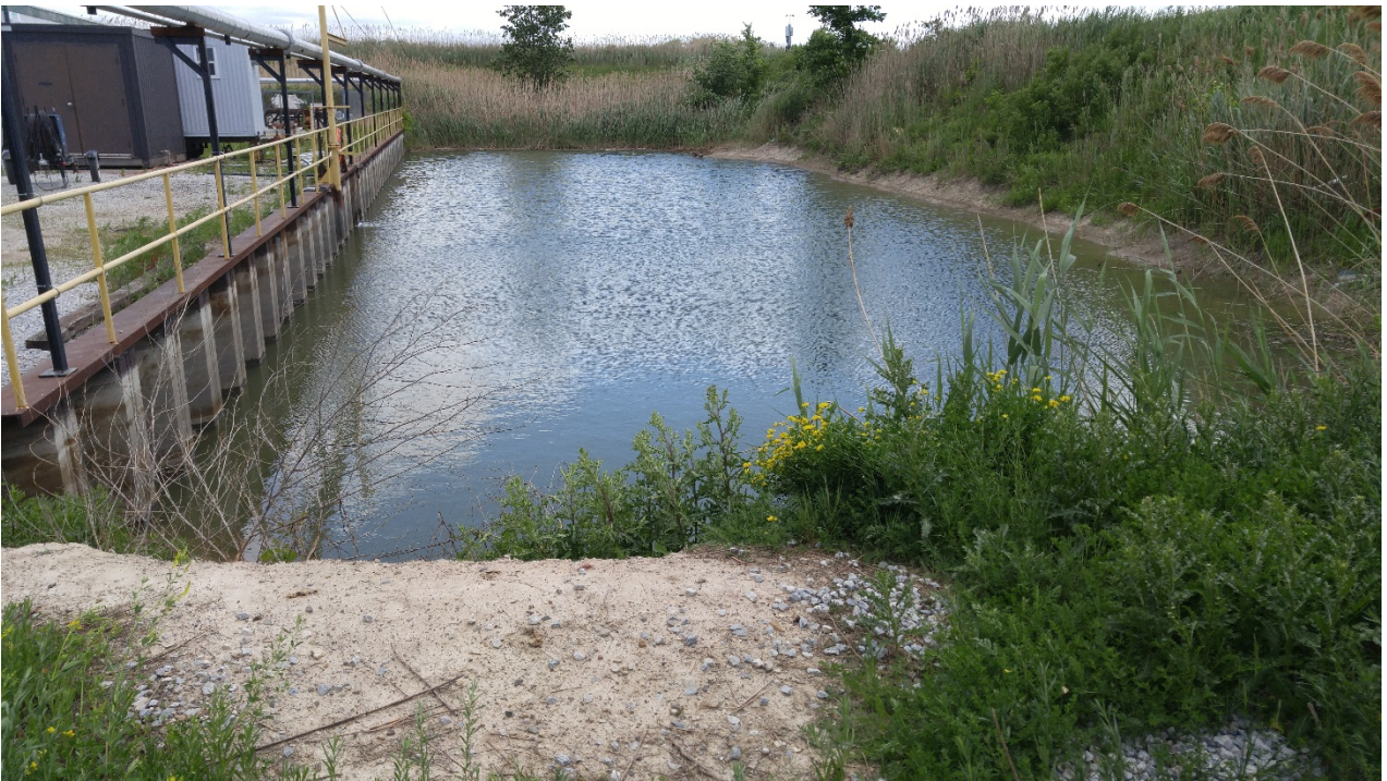
Photo 14 - South Process Water Pond
