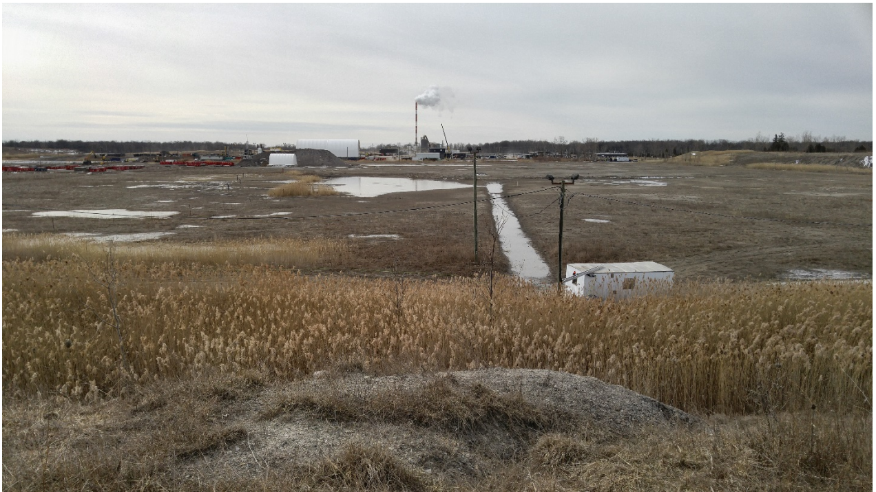
Photo 3 - Ponding within northwest corner of Site
