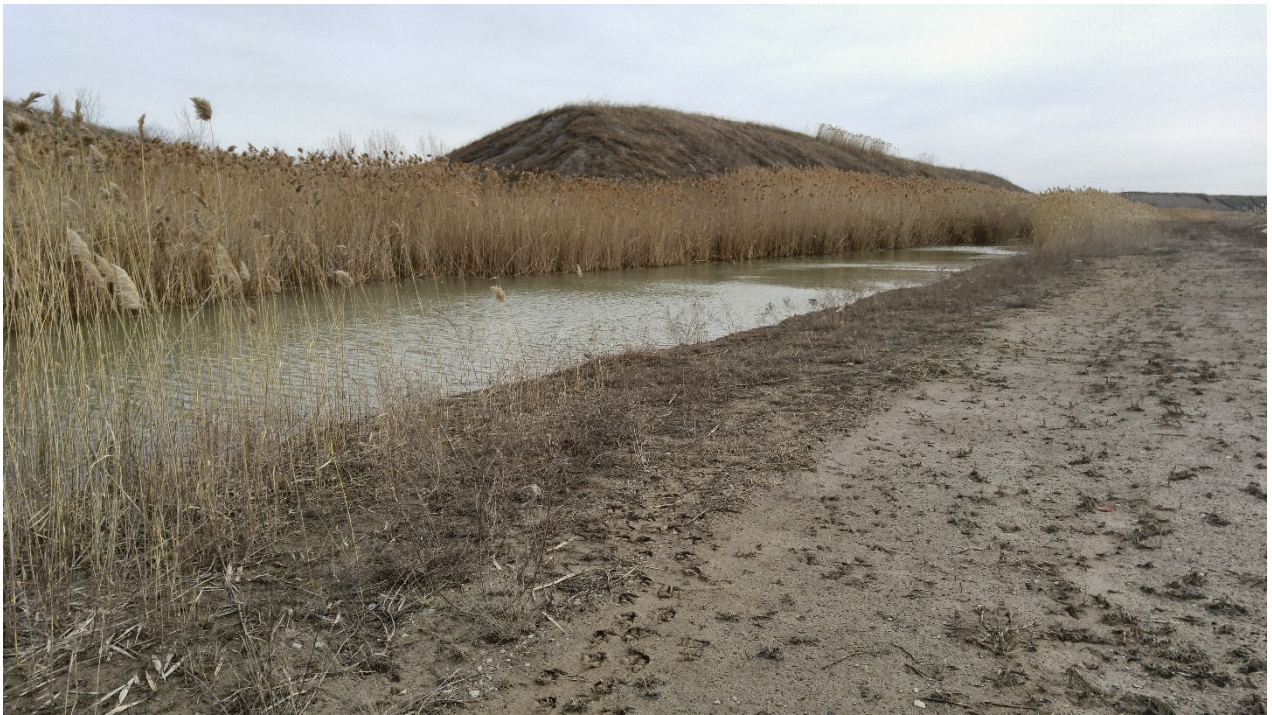
Photo 5 - High water levels in central portion of north perimeter ditch
