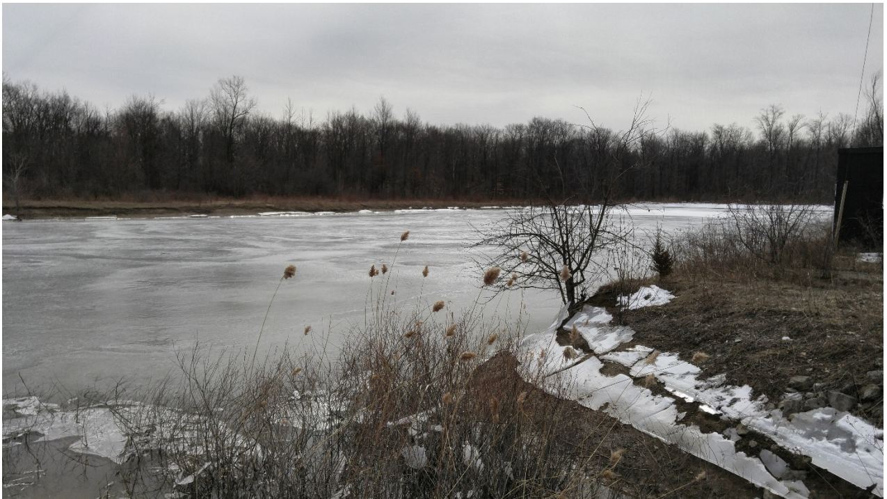
Photo 9 - East Surface Water Pond
