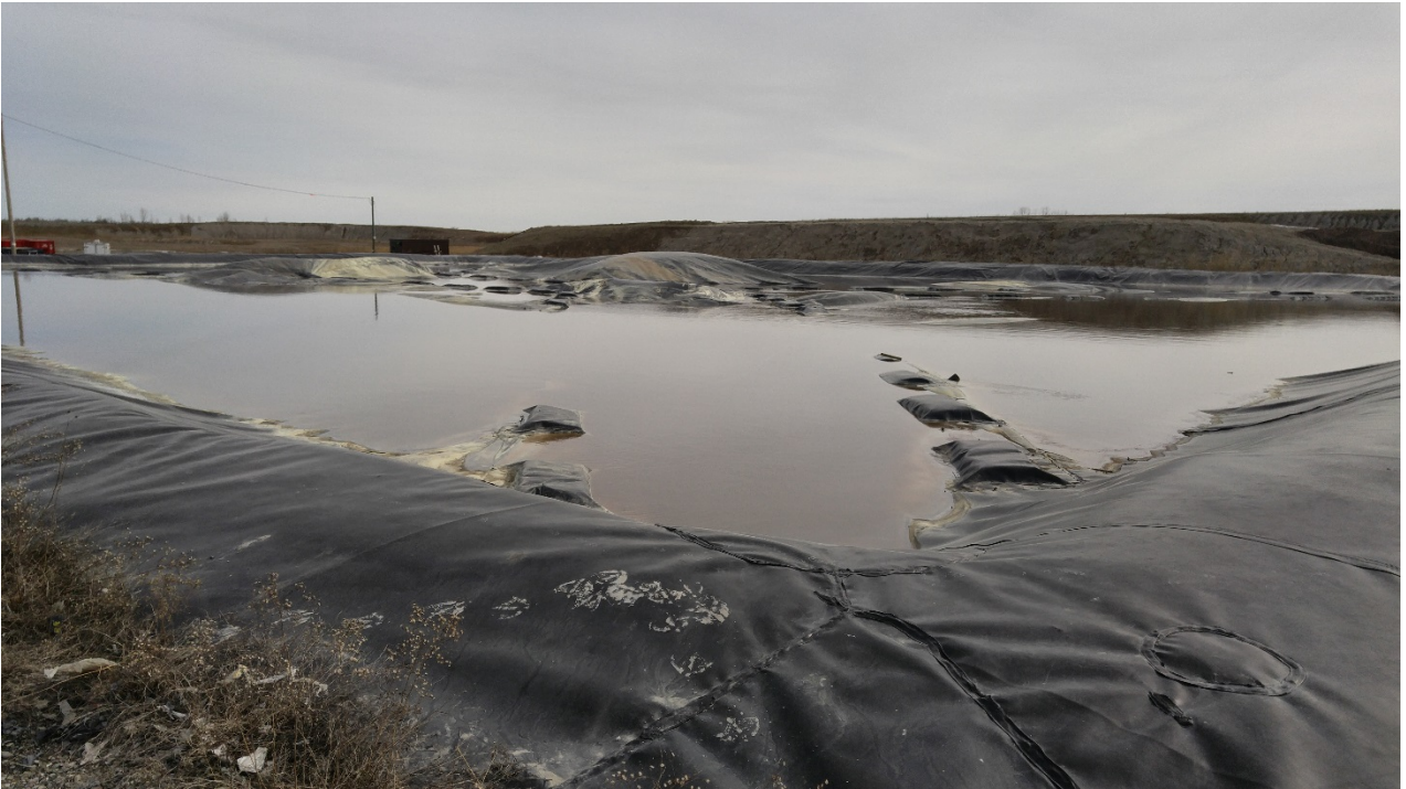
Photo 15 - East Leachate Reservoir
