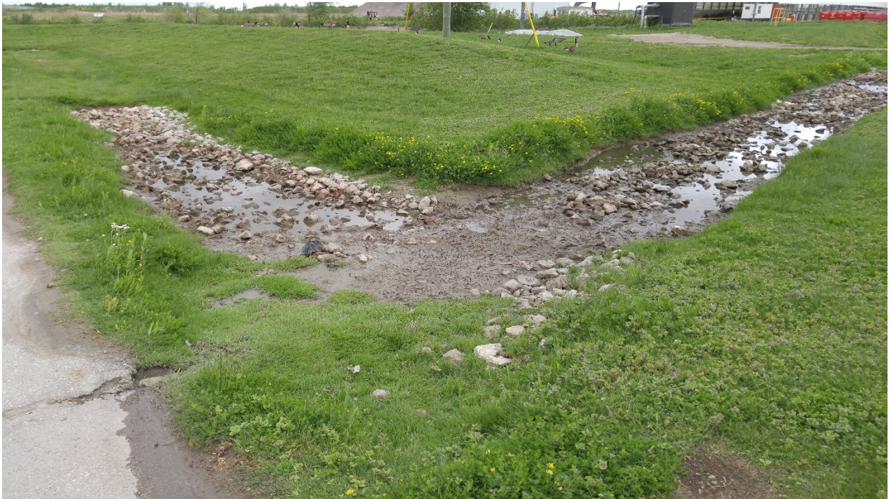
Photo 12 - North Process Water Pond ditch
