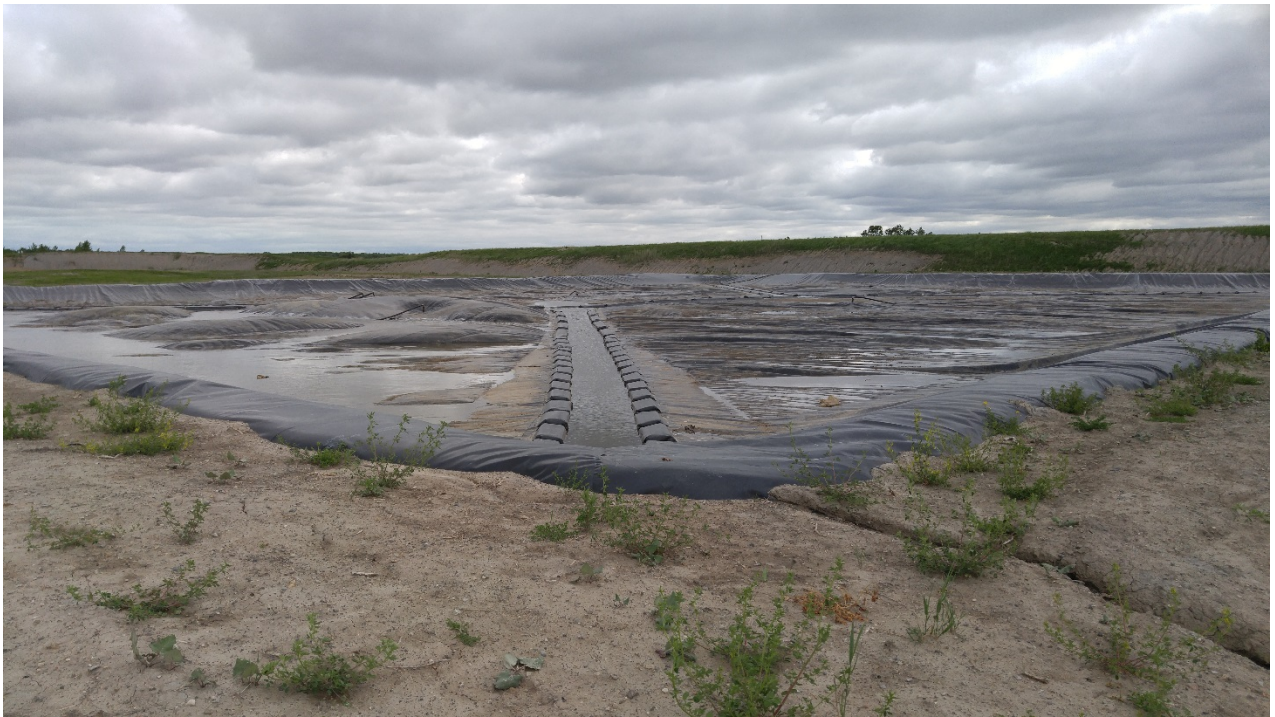
Photo 17 - New Leachate Reservoir
