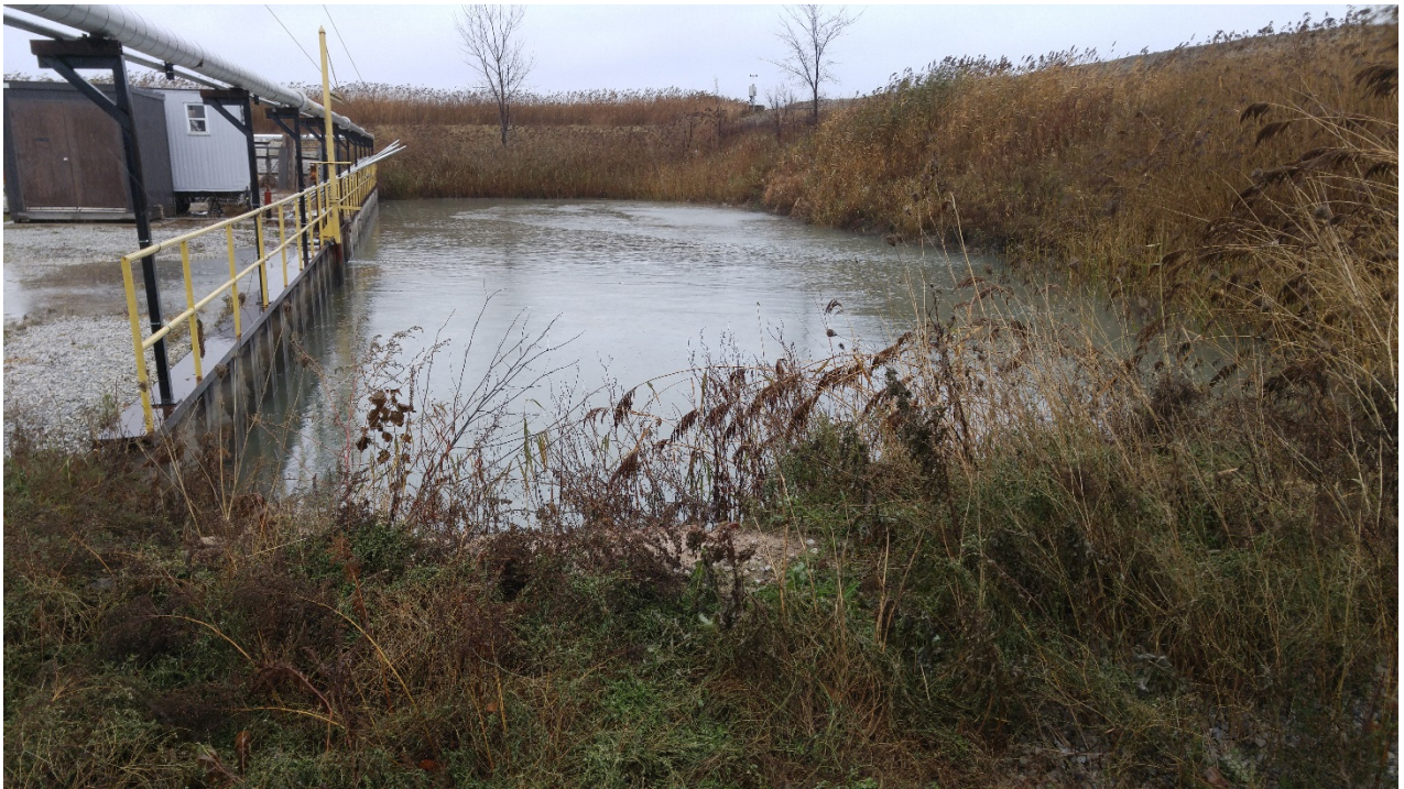
Photo 15 - South Process Water Pond
