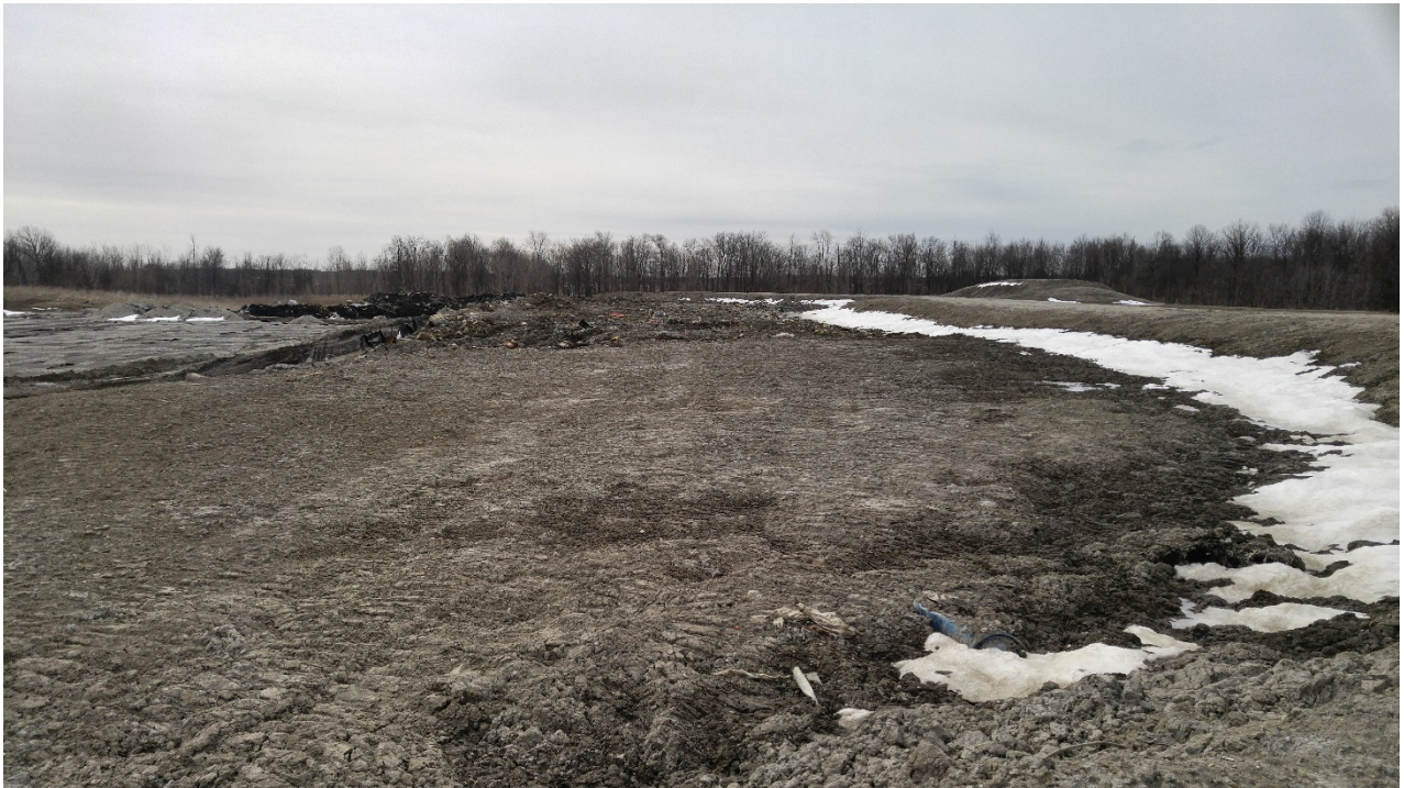
Photo 2 - Interim cap placement, southern portion of Cell 19-1-2
