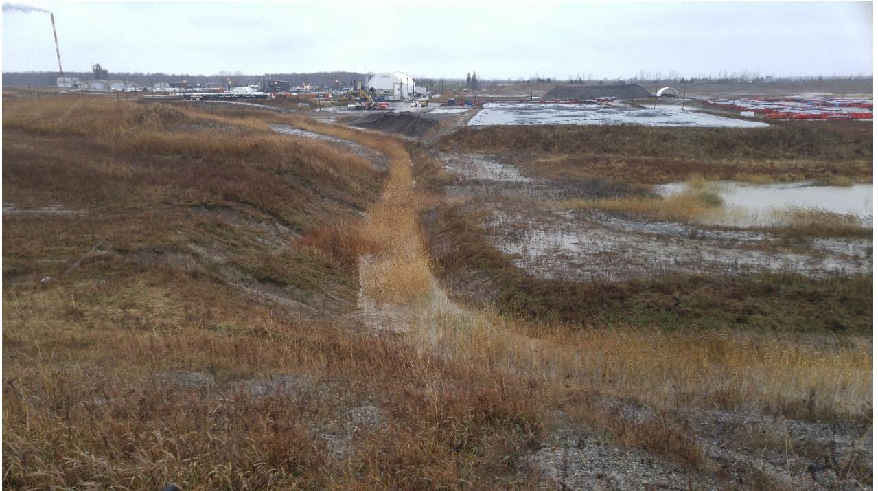
Photo 7 - North landfill area, southeast ditch, partial surface water blockage
