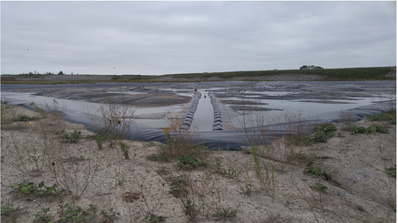
Photo 17 - New Leachate Reservoir
