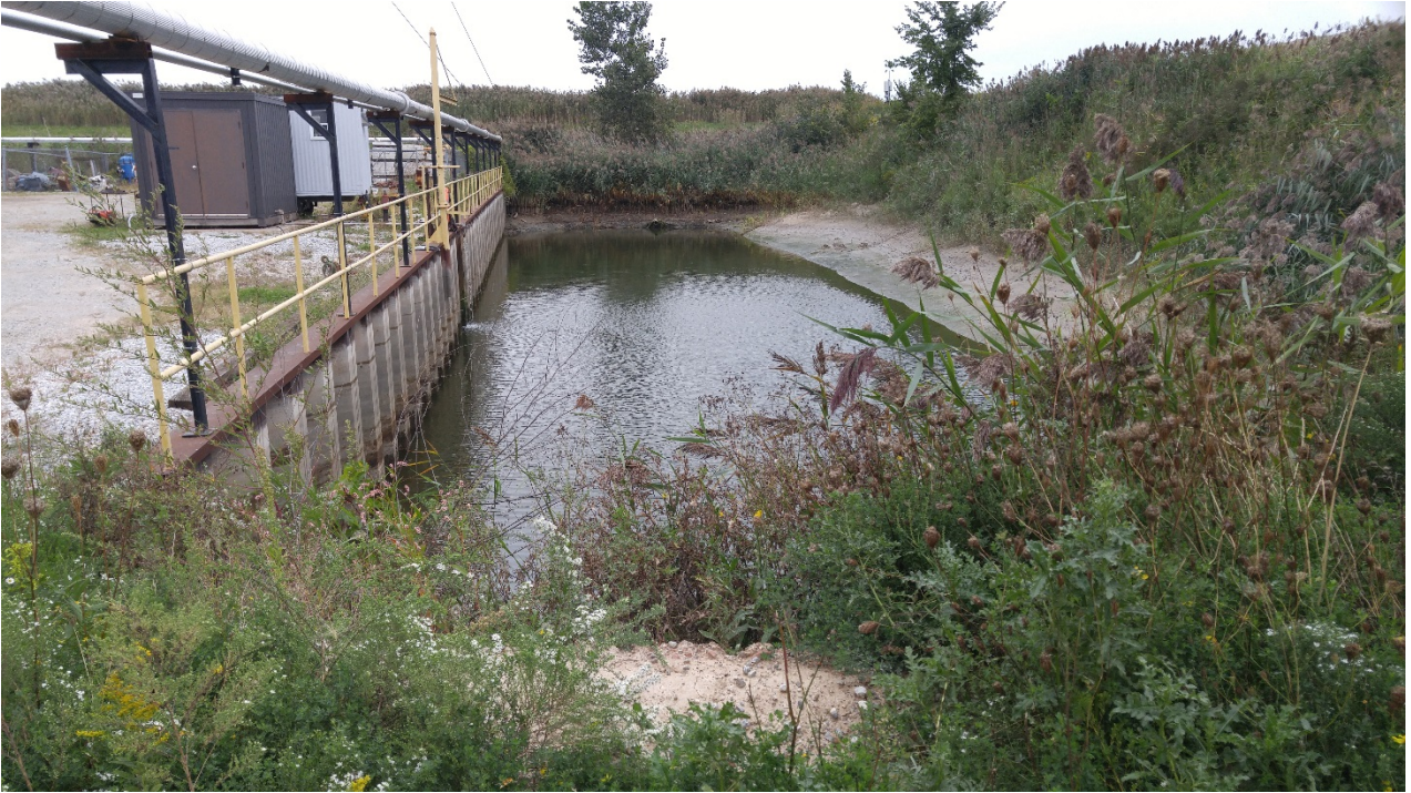
Photo 14 - South Process Water Pond
