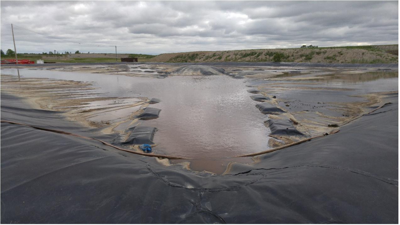
Photo 16 - East Leachate Reservoir
