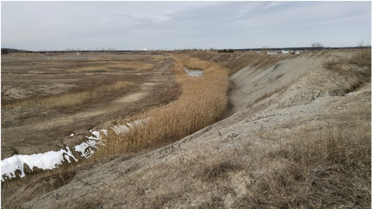
Photo 6 - North ditch, surface water blockage
