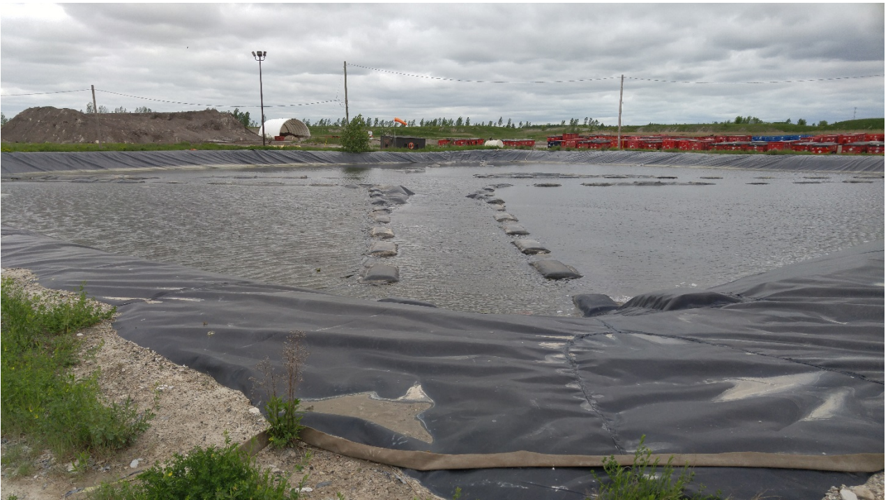
Photo 15 - South Leachate Reservoir
