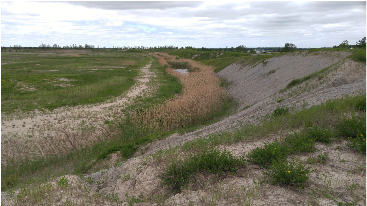
Photo 6 - North ditch, surface water blockage
