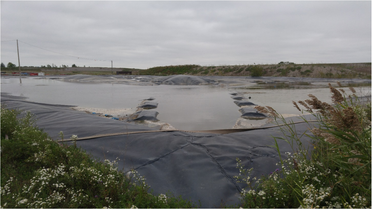
Photo 16 - East Leachate Reservoir
