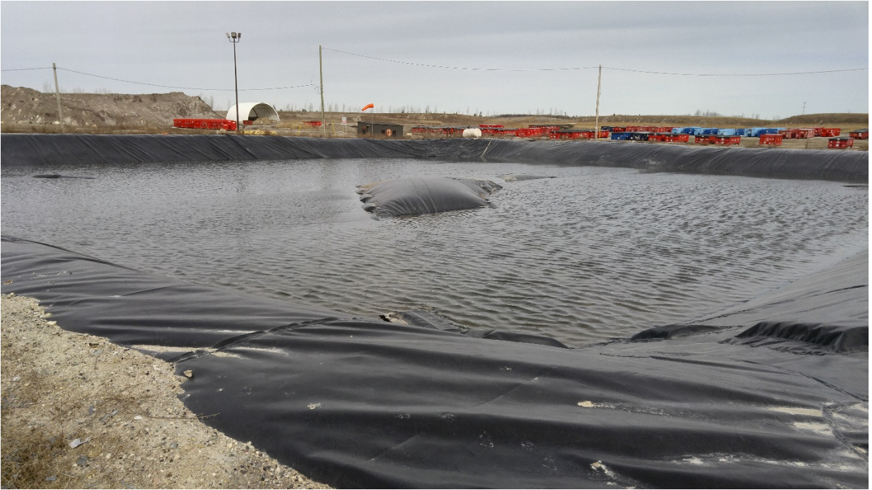
Photo 14 - South Leachate Reservoir
