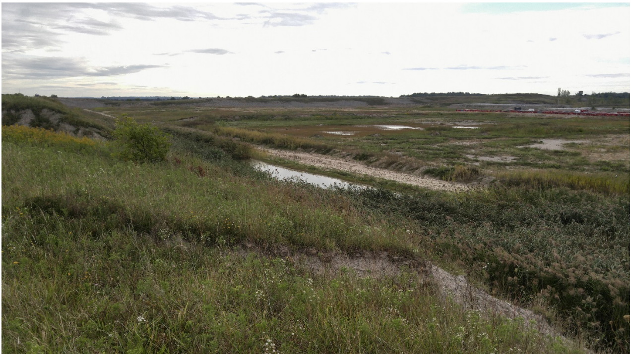
Photo 4 - Ponding in northern, central portion of Site
