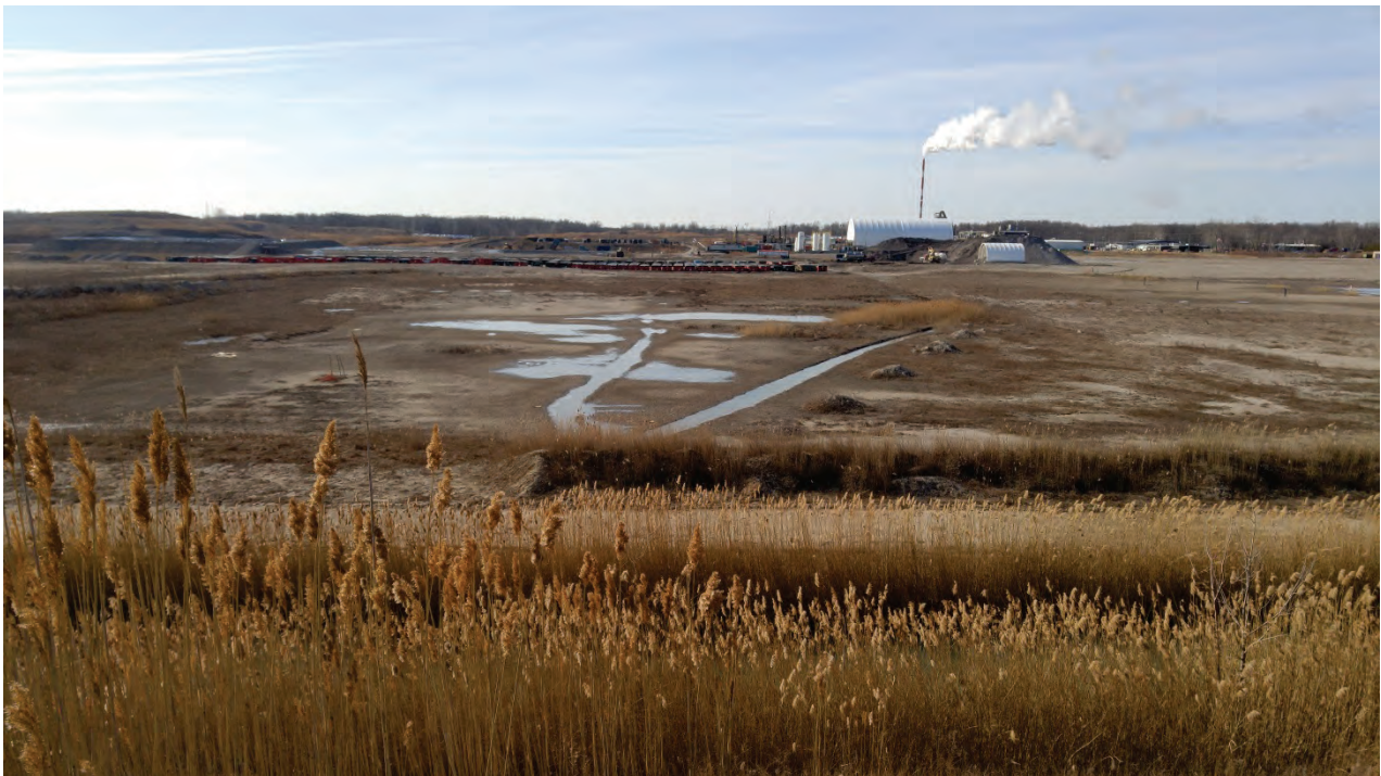
Photo 4 - Ponding in northern, central portion of Site
