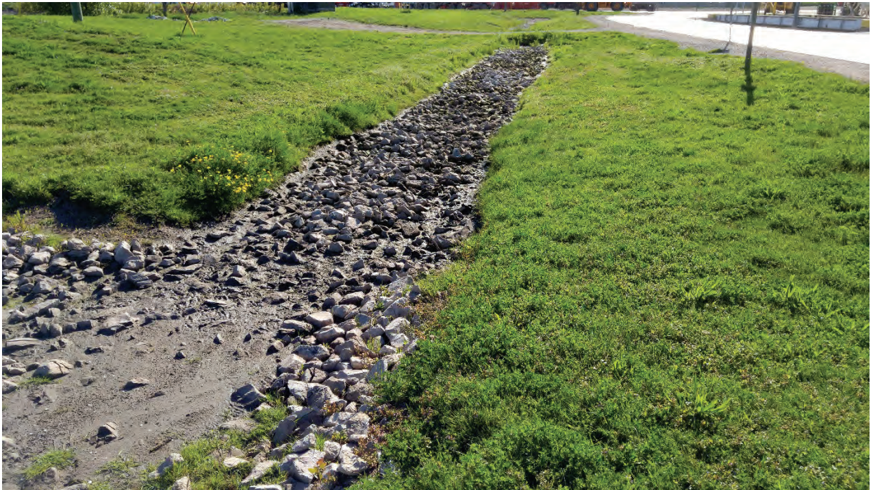
Photo 12 - North Process Water Pond ditch
