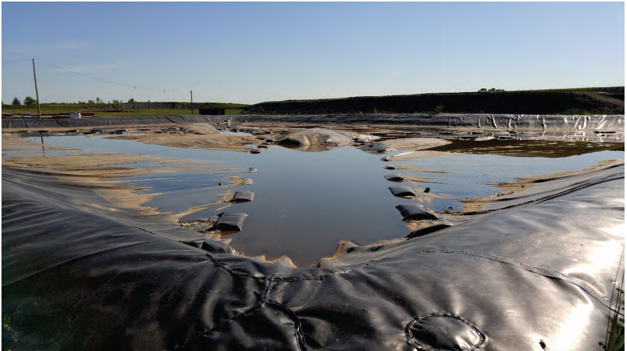
Photo 16 - East Leachate Reservoir
