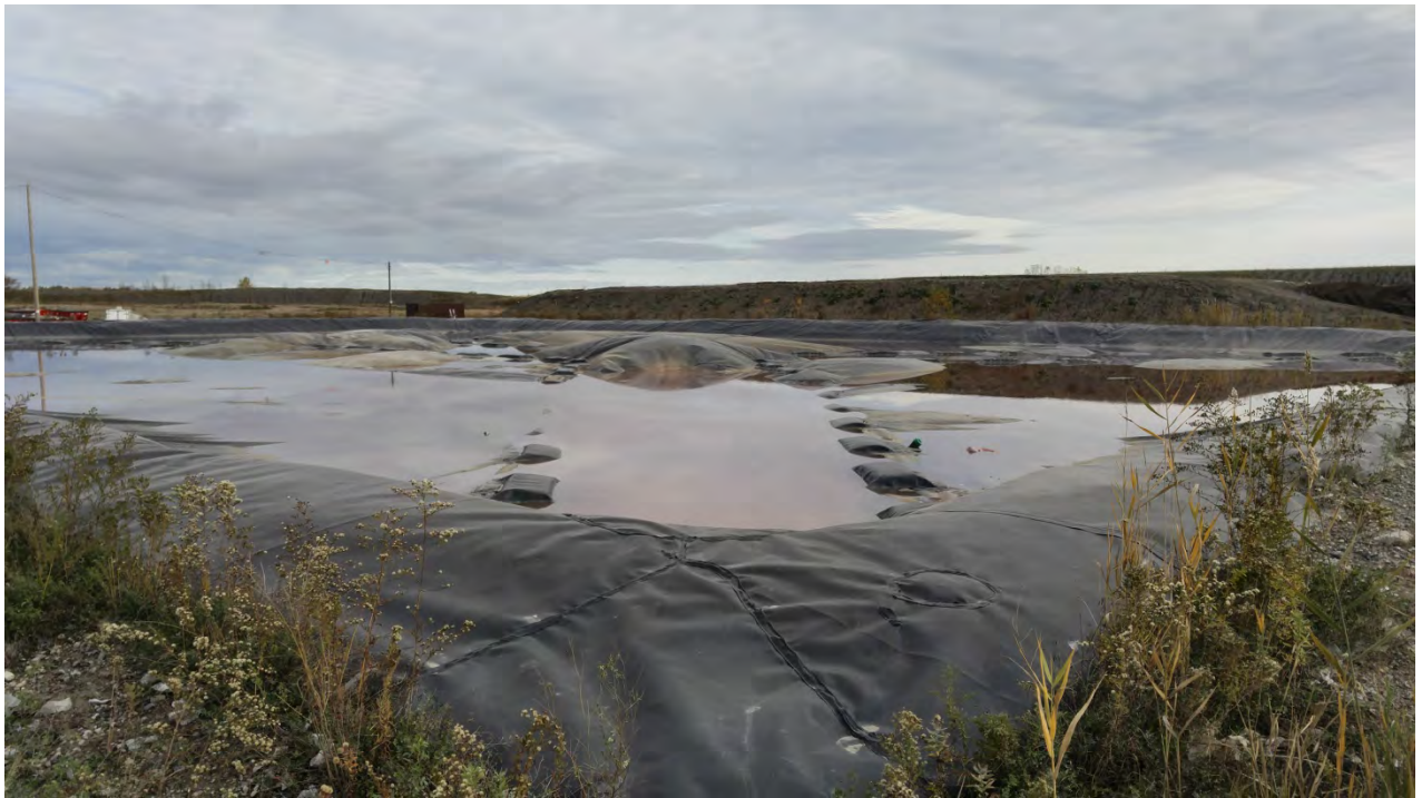
Photo 15 - East Leachate Reservoir
