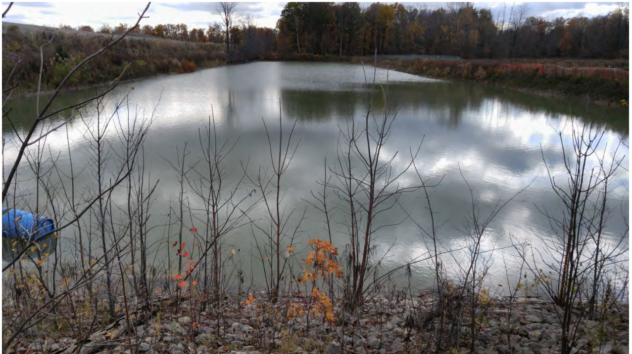
Photo 9 - West Surface Water Pond
