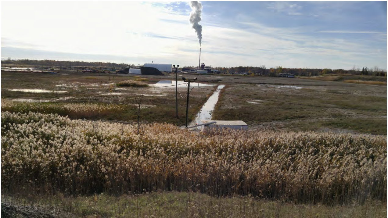
Photo 3 - Ponding within northwest corner of Site
