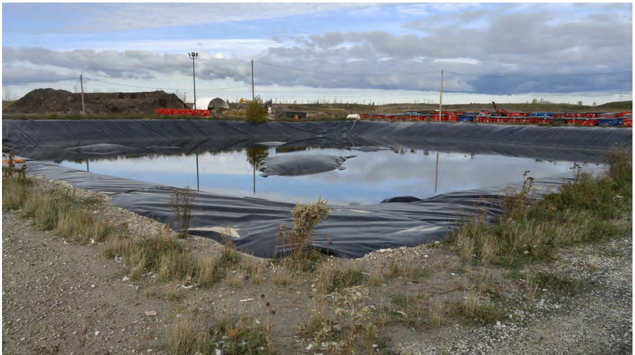
Photo 14 - South Leachate Reservoir
