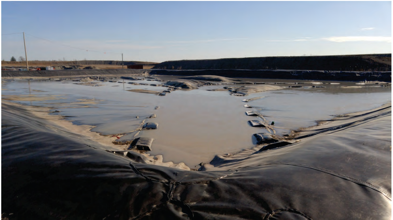
Photo 16 - East Leachate Reservoir
