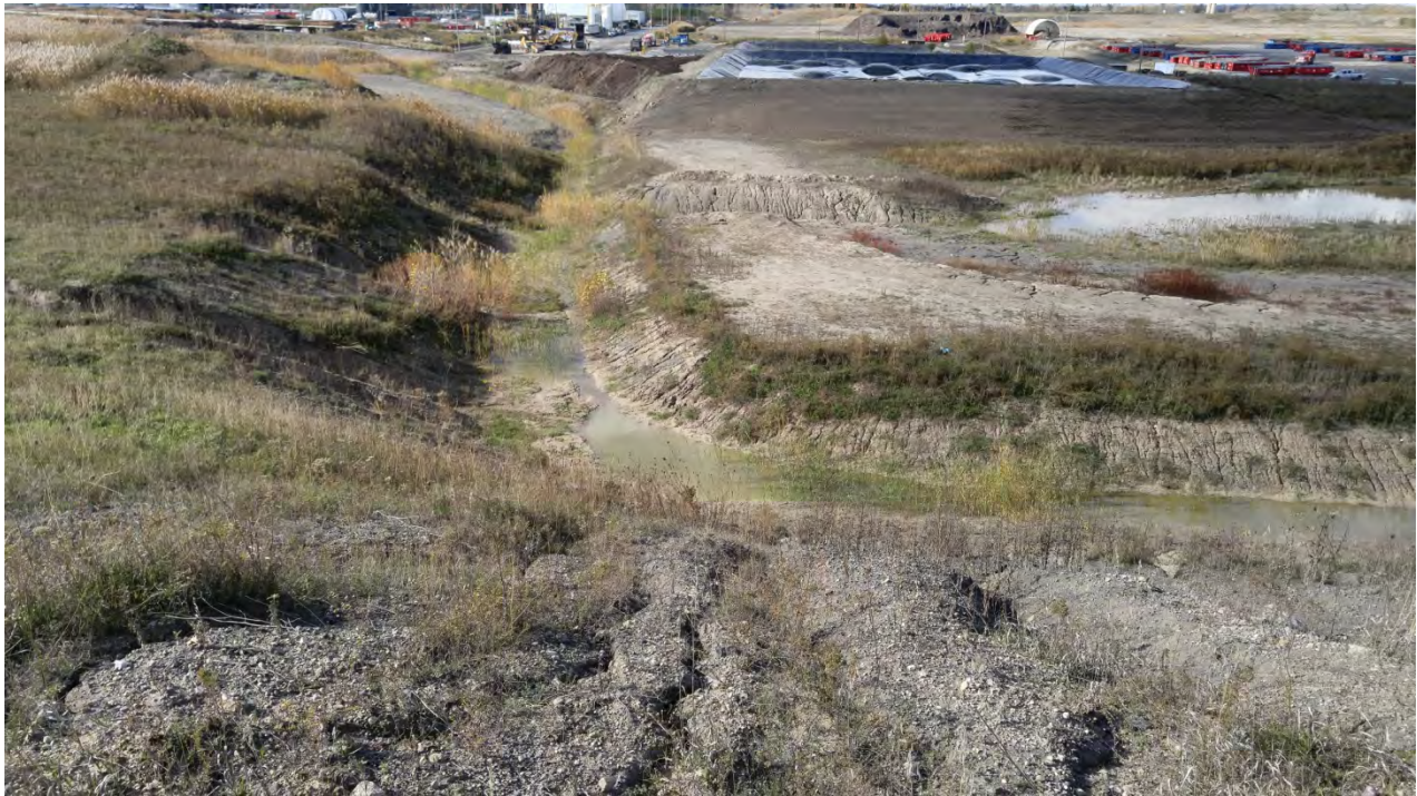
Photo 6 - North landfill area, southeast ditch, partial surface water blockage
