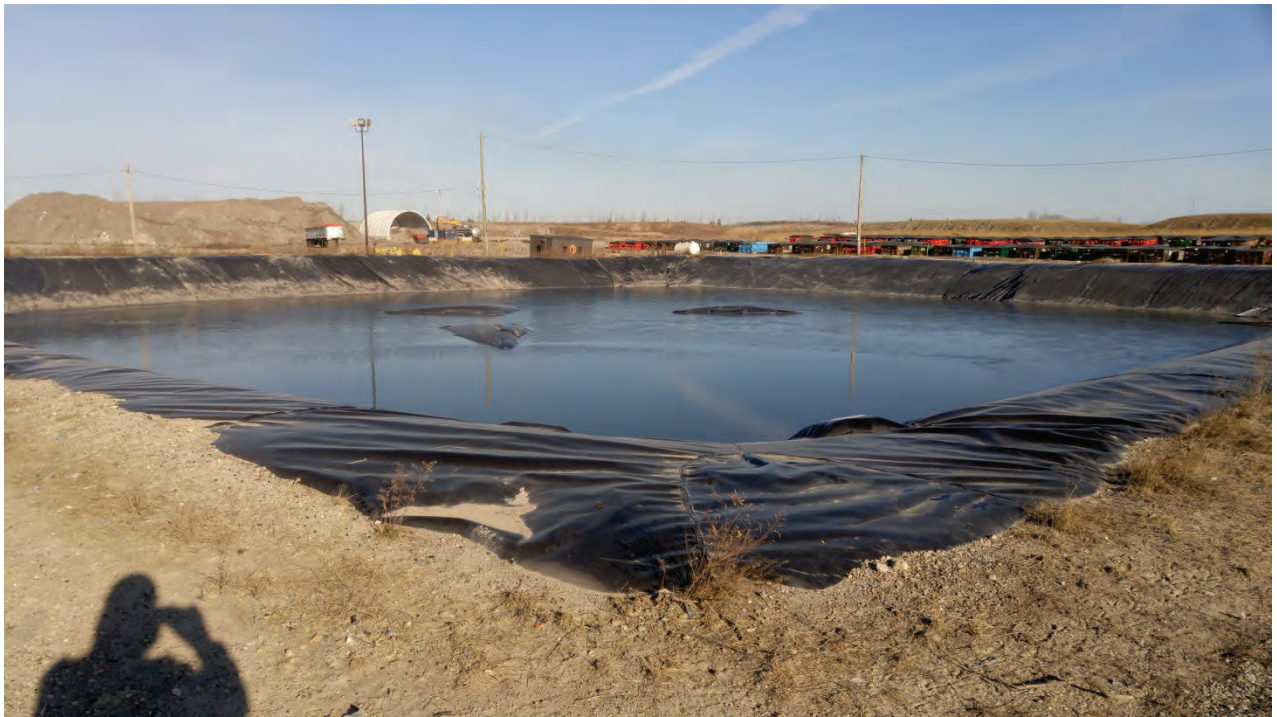
Photo 15 - South Leachate Reservoir
