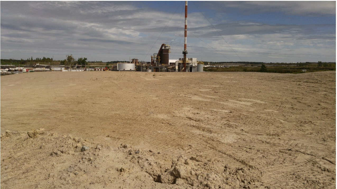
Photo 2 - Interim cap placement, southern portion of Cell 19-1-1
