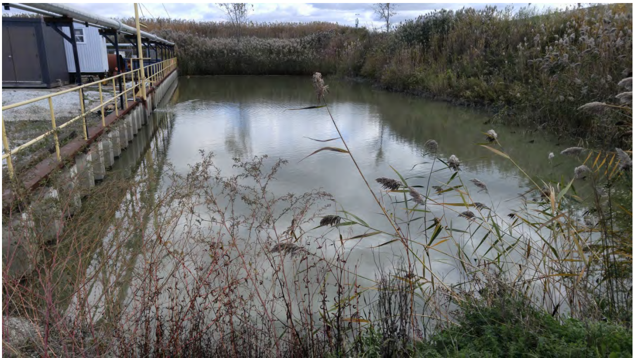
Photo 13 - South Process Water Pond
