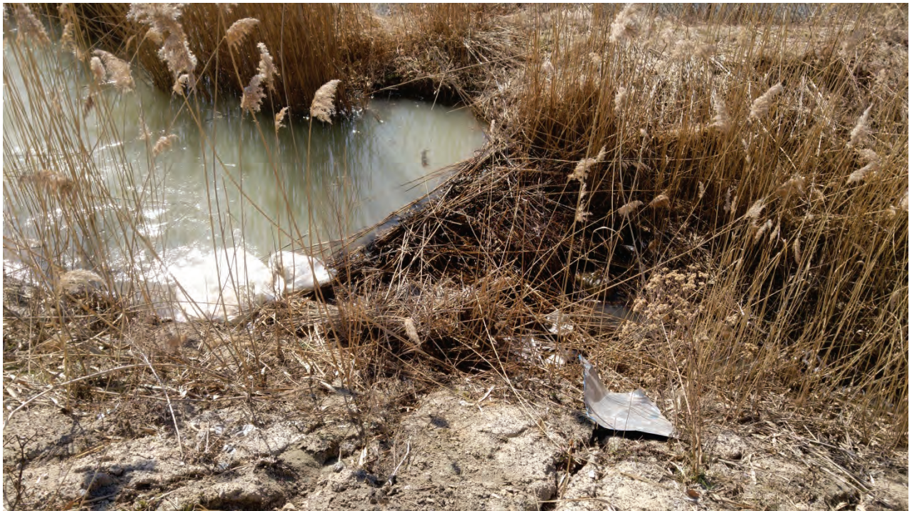
Photo 8 - Southwest ditch, surface water blockage
