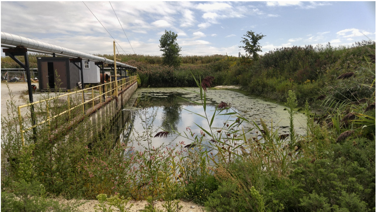
Photo 13 - South Process Water Pond
