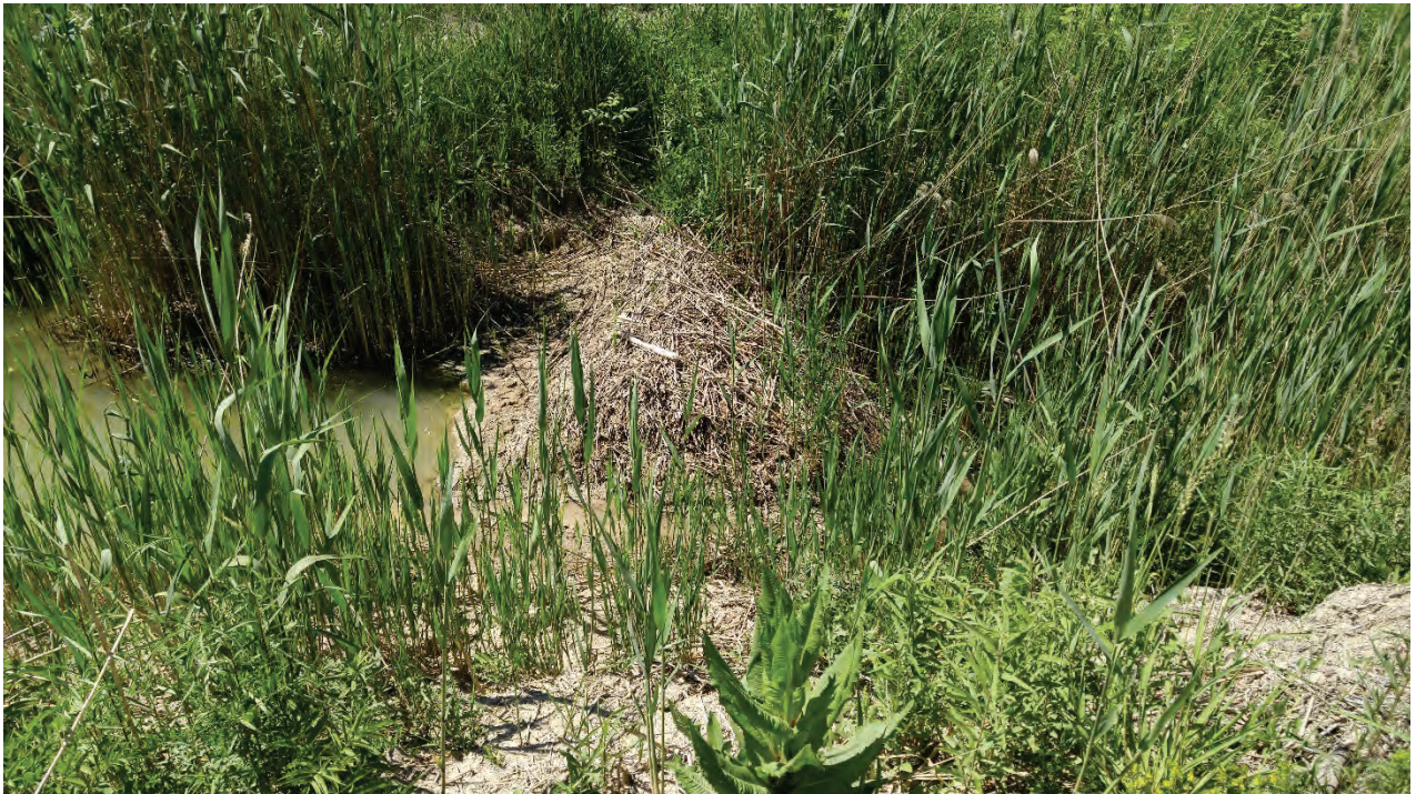
Photo 8 - Southwest ditch, surface water blockage
