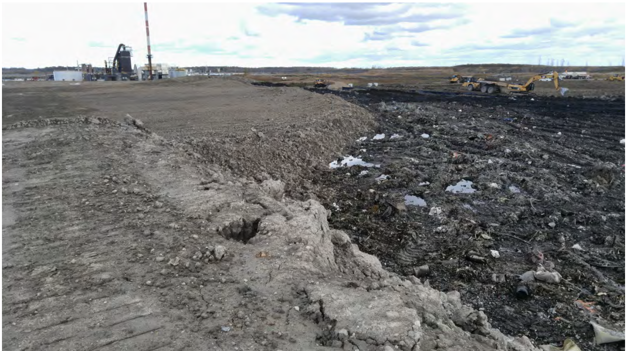
Photo 2 - Interim cap placement, southern portion of Cells 19-1-1 and 19-1-2
