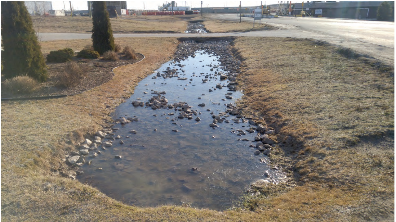
Photo 12 - North Process Water Pond ditch
