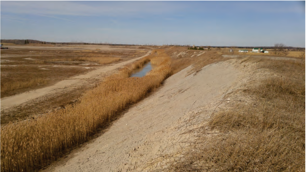
Photo 5 - North ditch, surface water blockage
