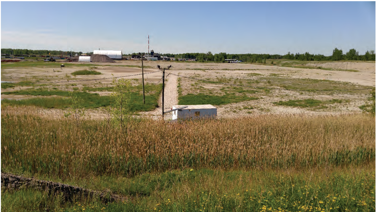
Photo 3 - Ponding within northwest corner of Site
