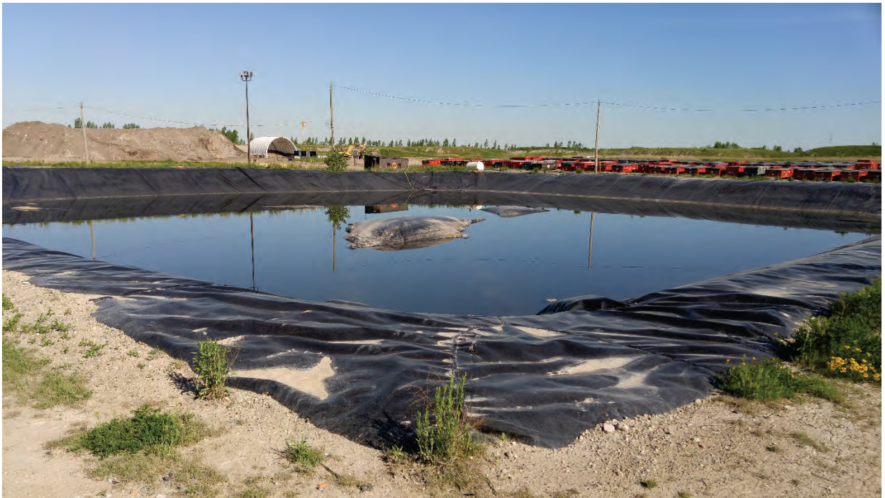
Photo 15 - South Leachate Reservoir
