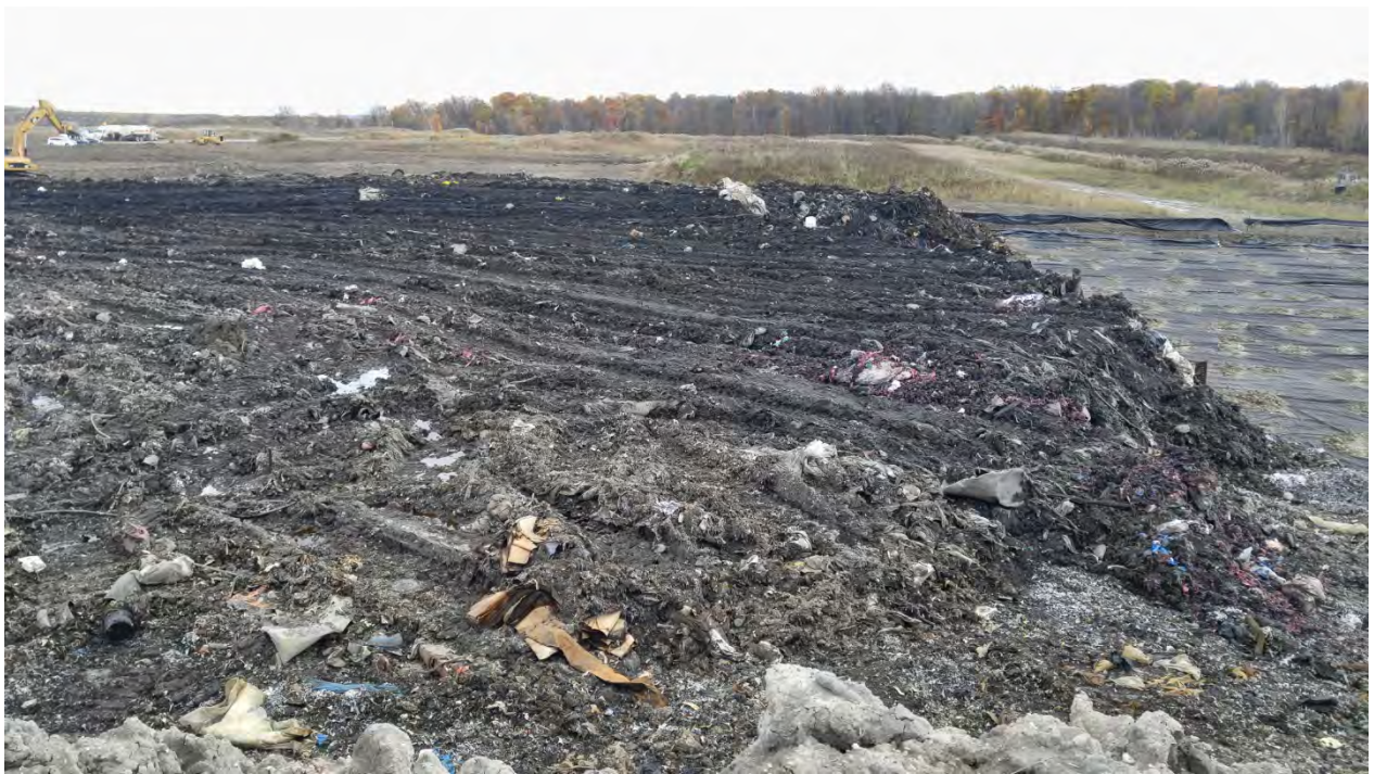
Photo 1 - Active landfilling cell (southern portion of Cell 19-1-2)
