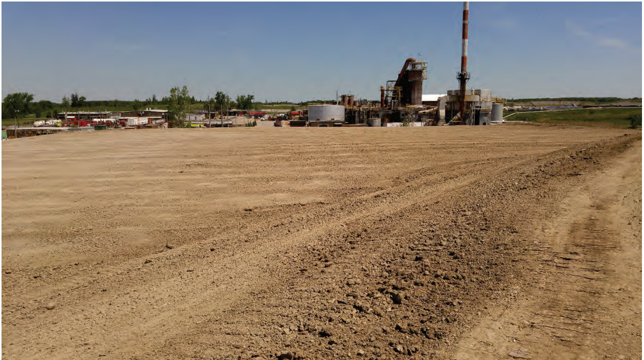
Photo 2 - Interim cap placement, southern portion of Cell 19-1-1
