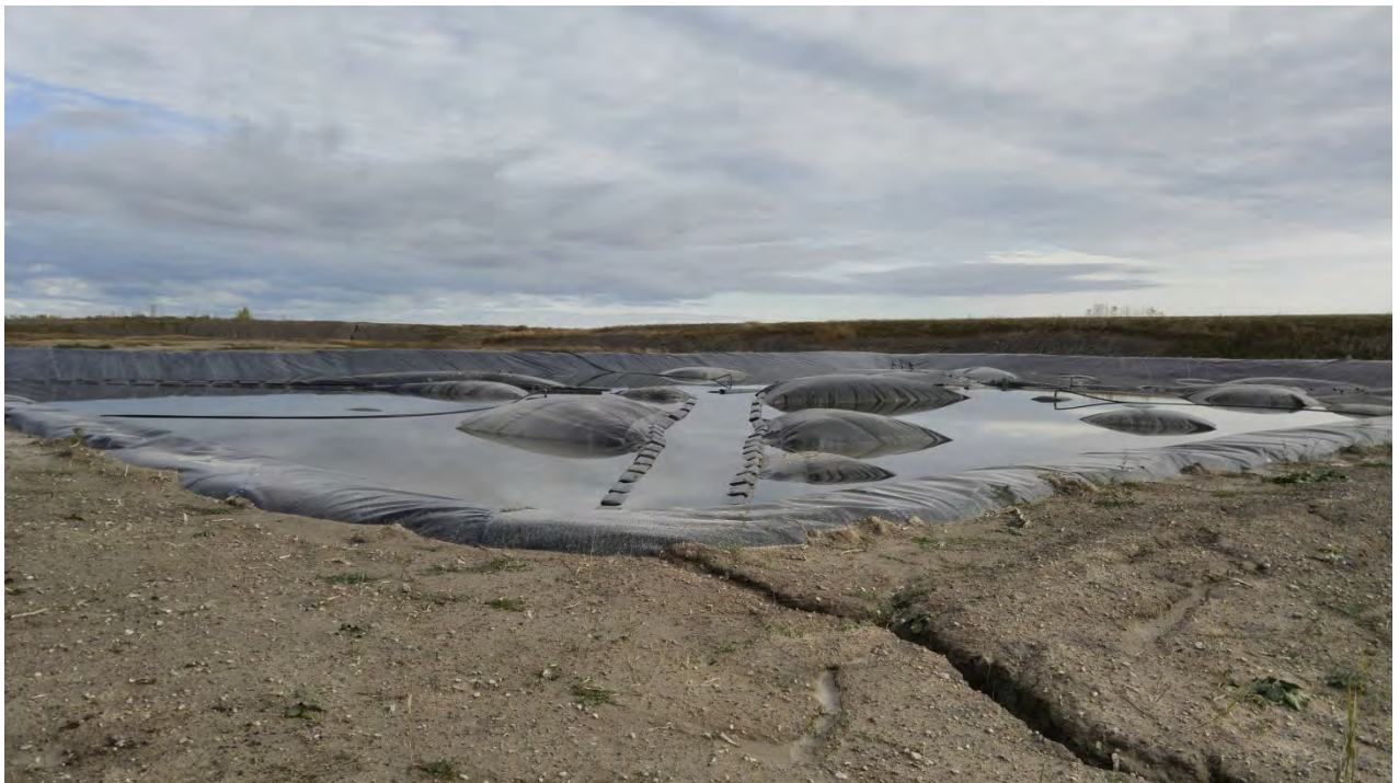
Photo 16 - New Leachate Reservoir
