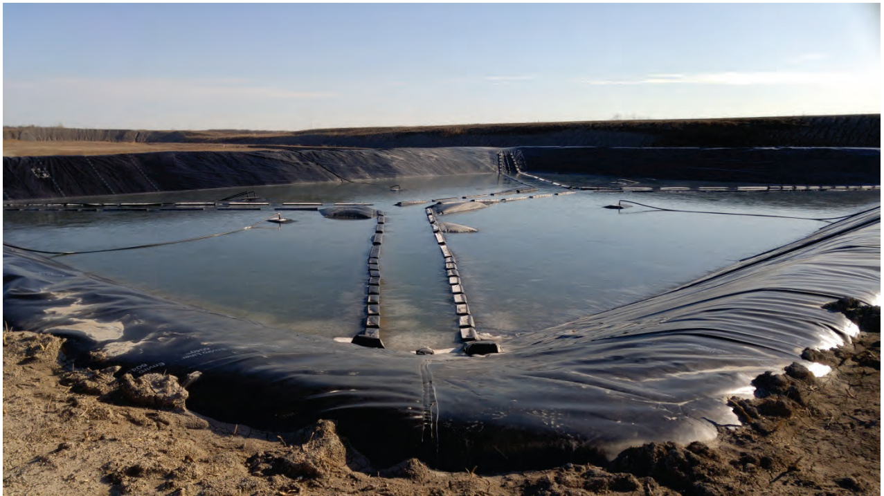
Photo 17 - Newly Constructed Leachate Reservoir
