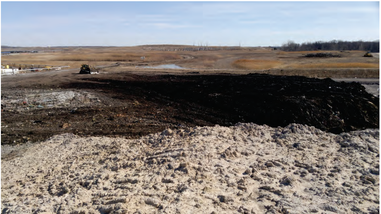
Photo 1 - Active landfilling cell (northern portion of Cell 19-1-2)
