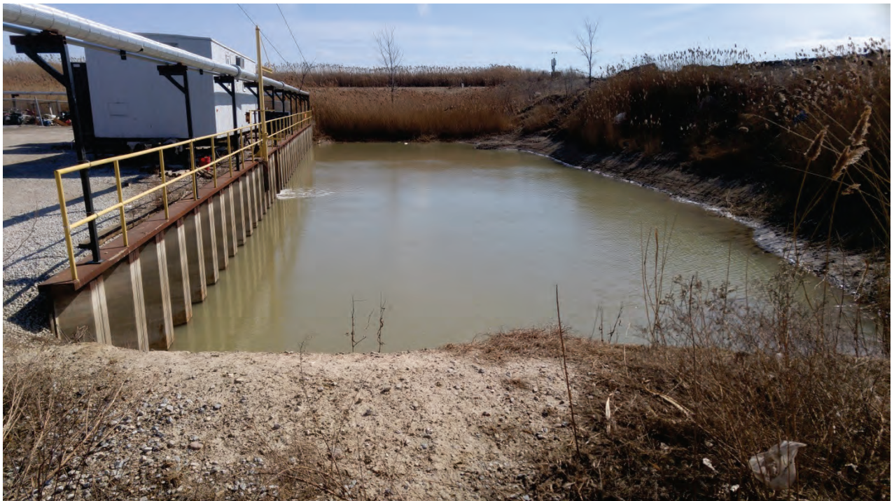
Photo 14 - South Process Water Pond
