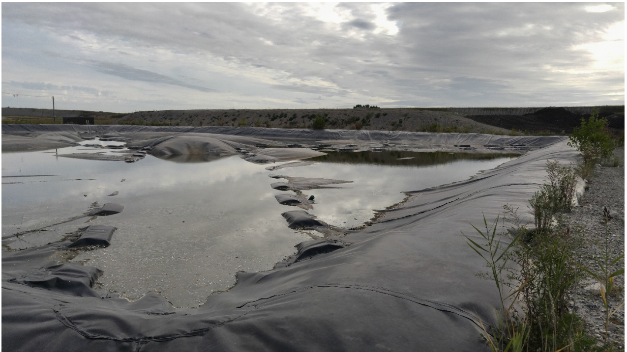
Photo 15 - East Leachate Reservoir
