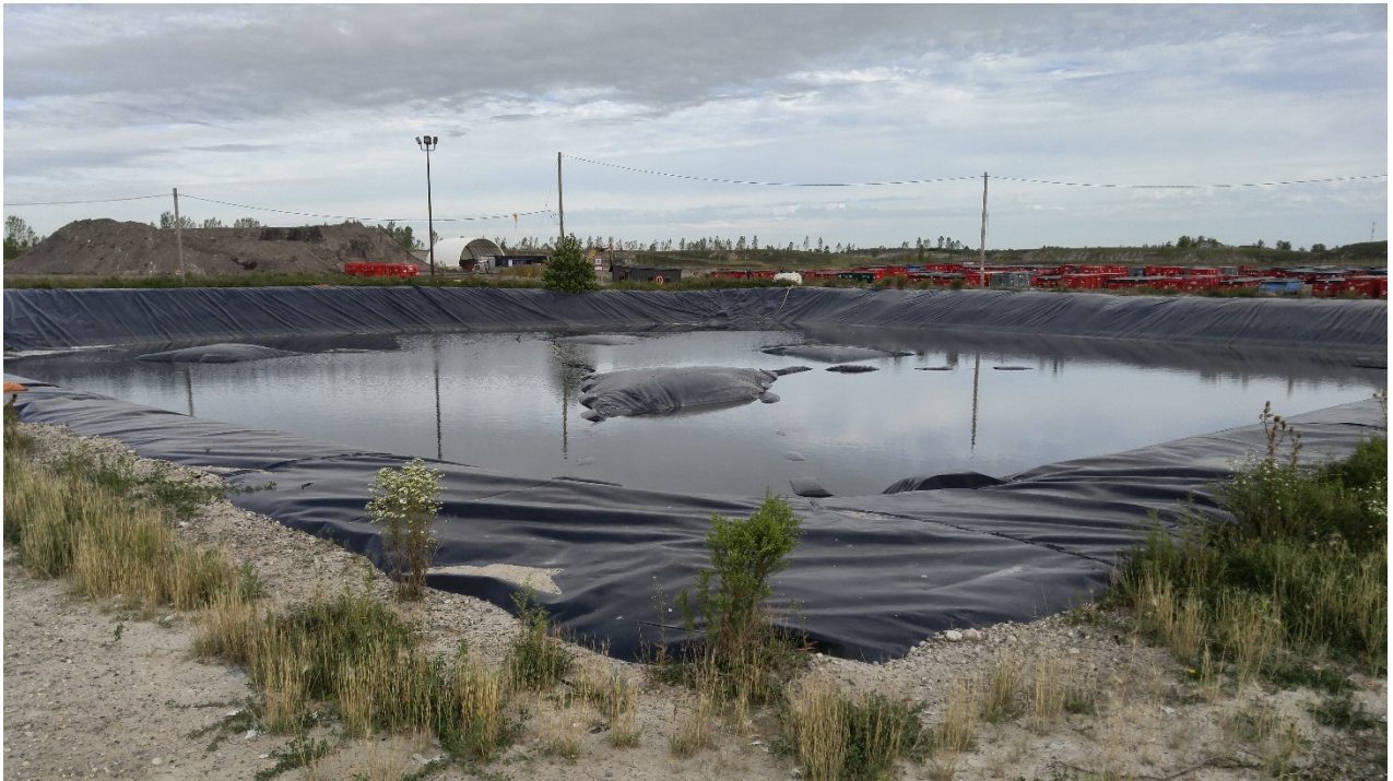
Photo 14 - South Leachate Reservoir
