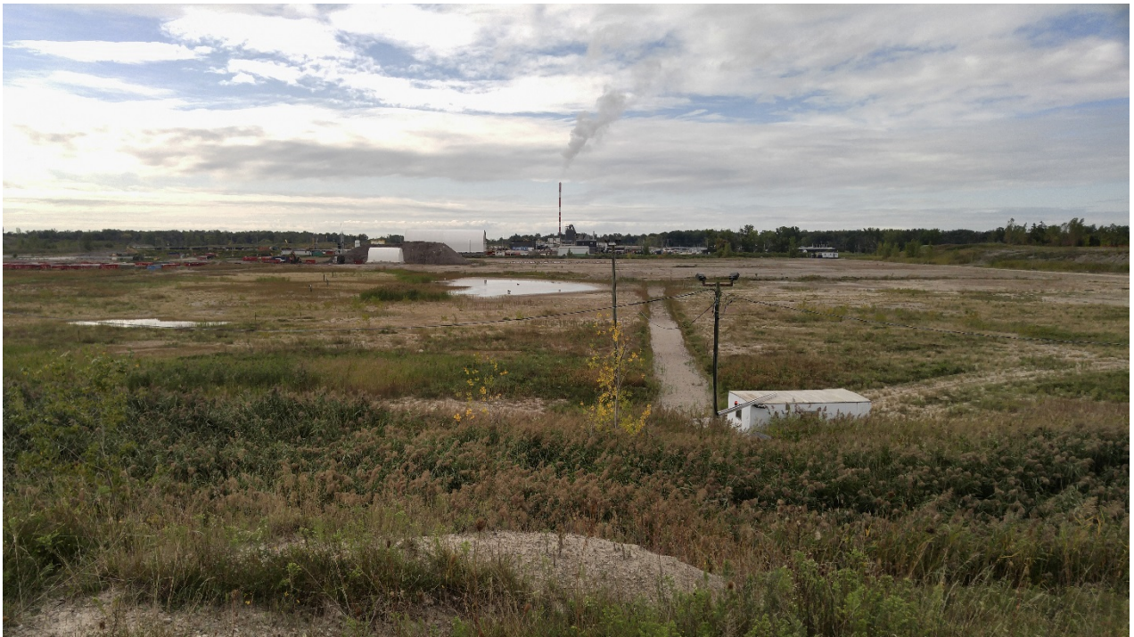
Photo 3 - Ponding within northwest corner of Site
