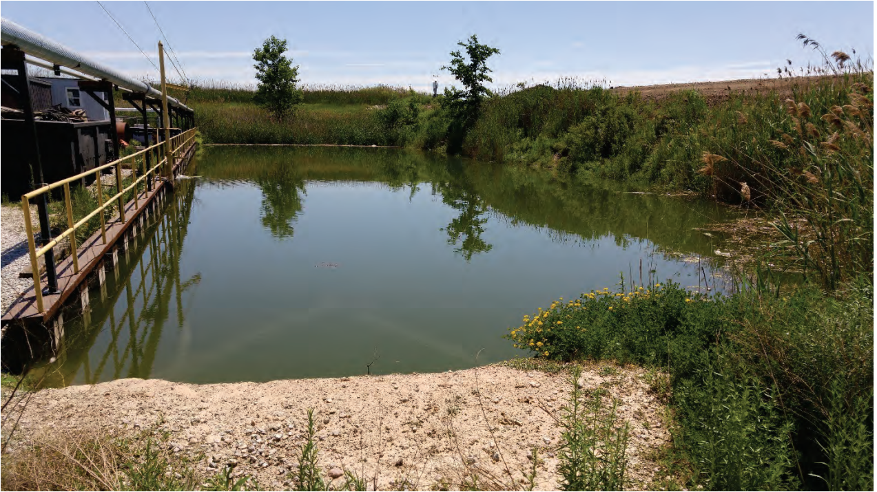
Photo 14 - South Process Water Pond
