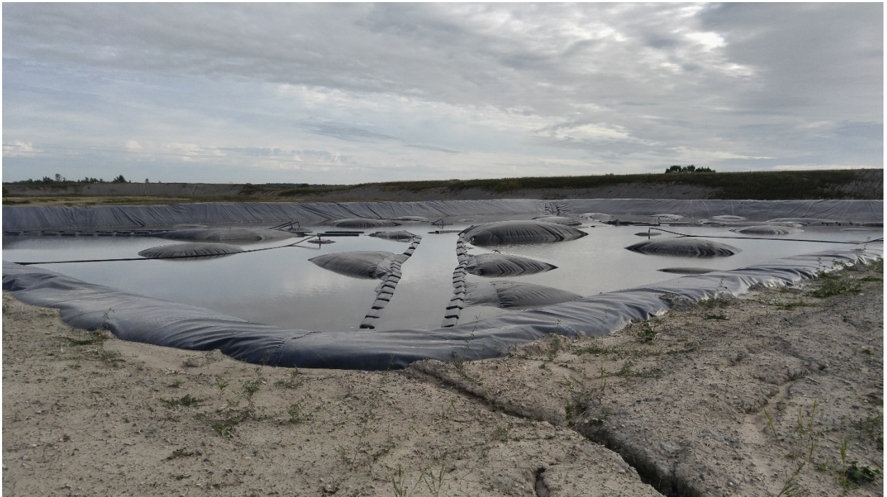
Photo 16 - New Leachate Reservoir
