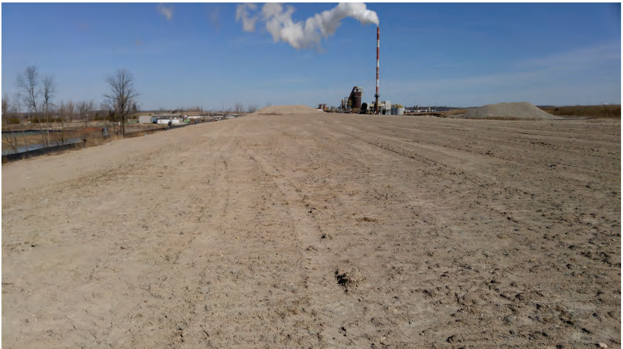
Photo 2 - Interim cap placement, southern portion of Cell 19-1-1
