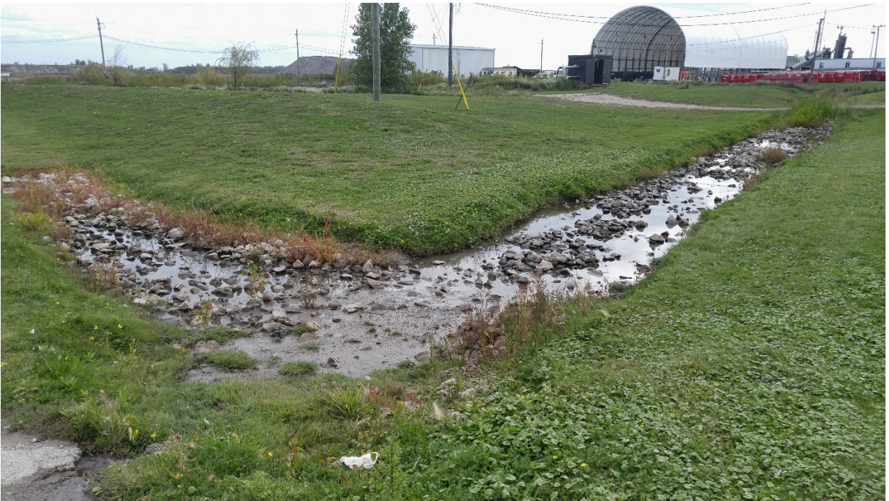
Photo 11 - North Process Water Pond ditch
